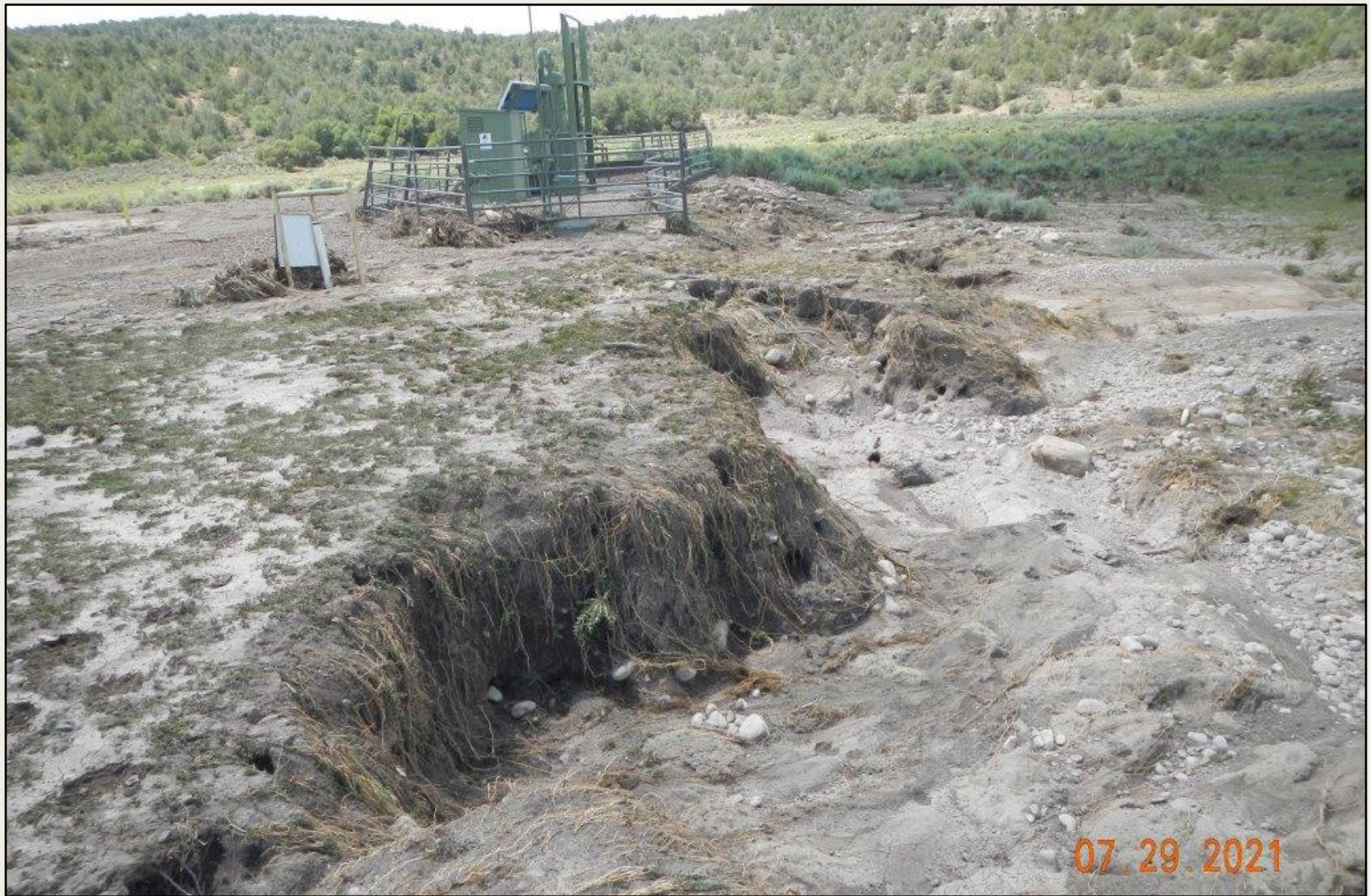
Photo 1. View of the location from the northwestern corner facing southward. Flood event has washed well pad material off of well pad and deposited down-slope and downstream. Water flow is from right to left here.
