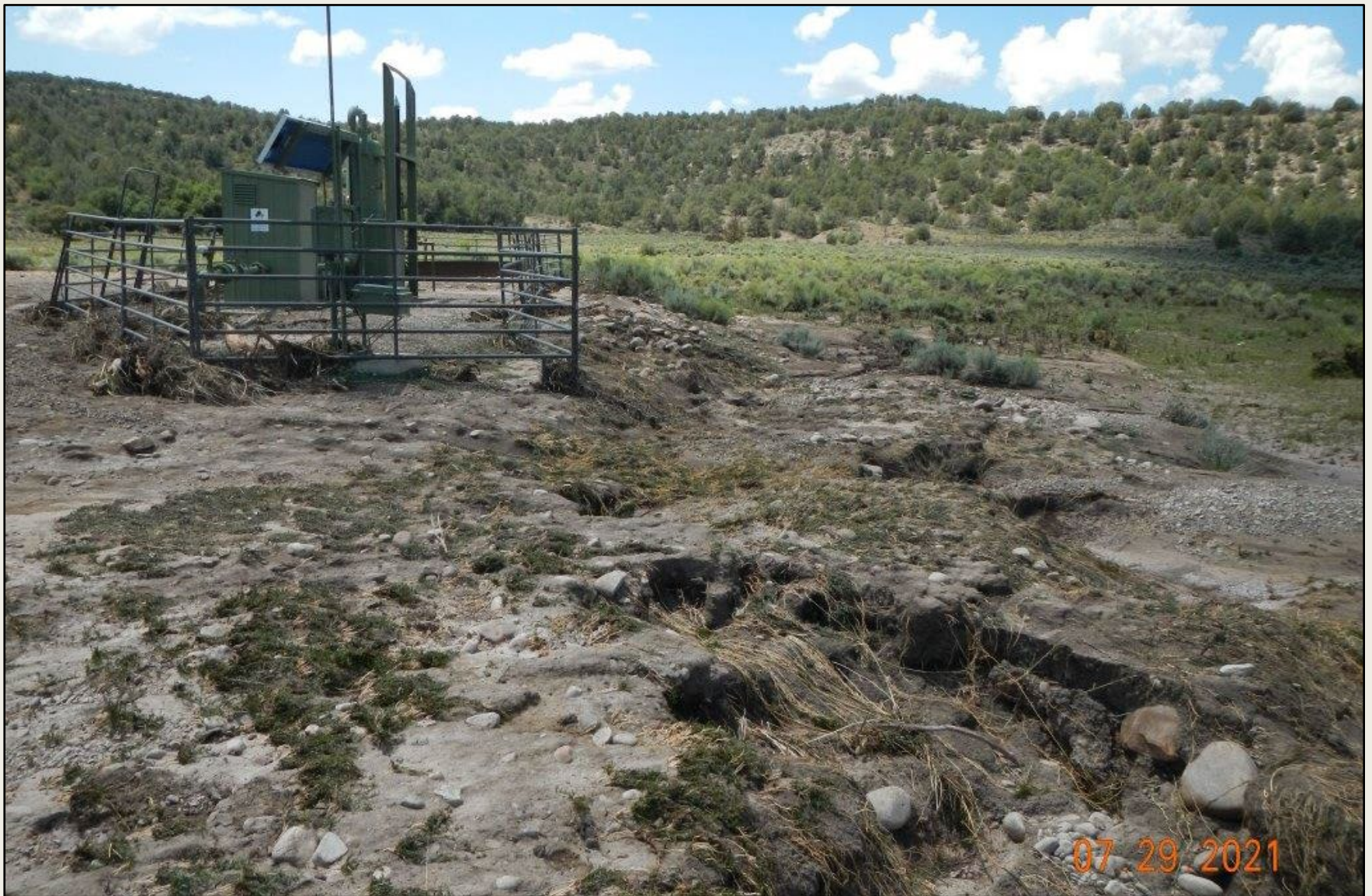
Photo 2. View of area where flood water has washed away well pad material, and deposited wood and plant debris on project facilities.
