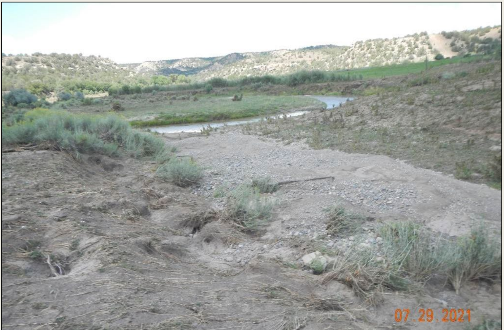
Photo 4. View of a high volume of well pad material discharging off of the project area into the river and along the banks of the river (facing downstream).
