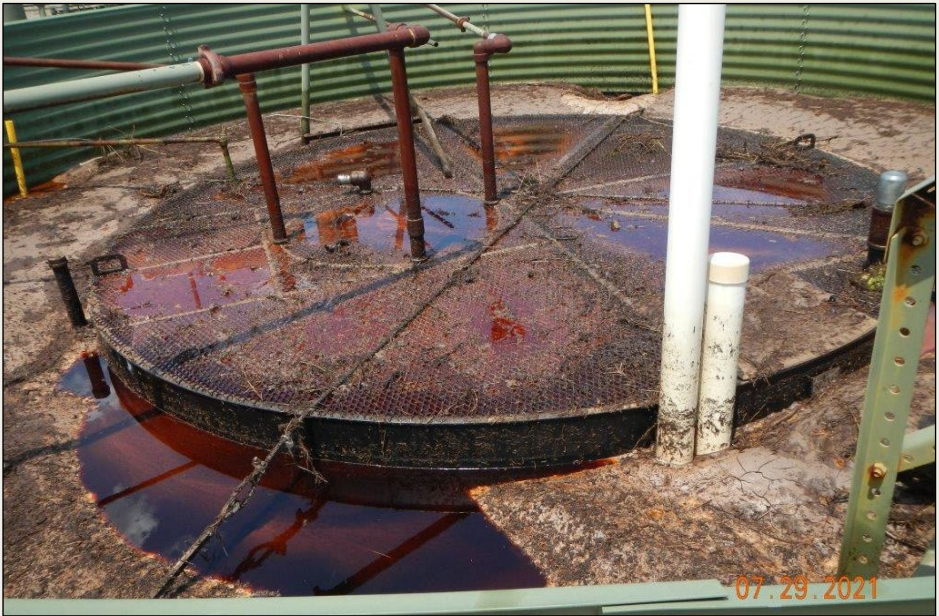
Photo 10. View of tank overflowing in eastern portion of the project area. Oily material pooled outside of tank. Wood debris deposited within and on top of tank.
