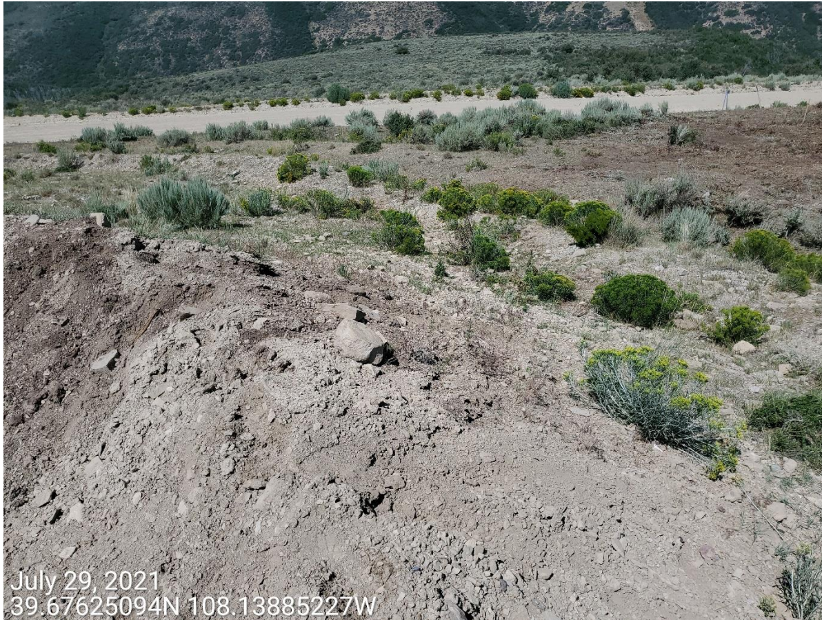
Photo 3: Photo taken from the north end of the Location, facing west. Photo shows slopes that remain loose material at risk to erosion; control measures to protect and stabilize slopes remain missing or insufficient.
