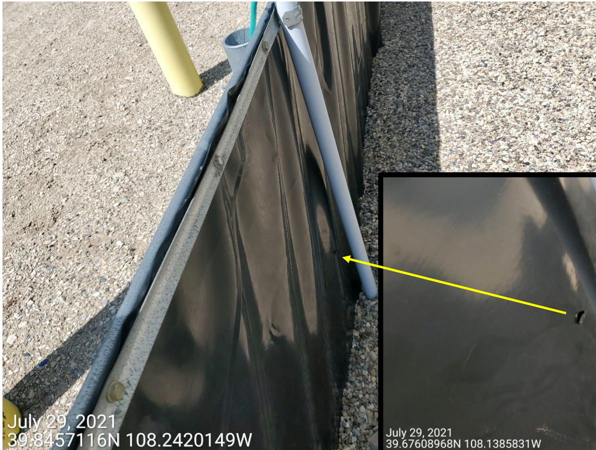
Photo 2: Photo taken from the liner on the south end of the tank battery. Photo shows tear in liner.
