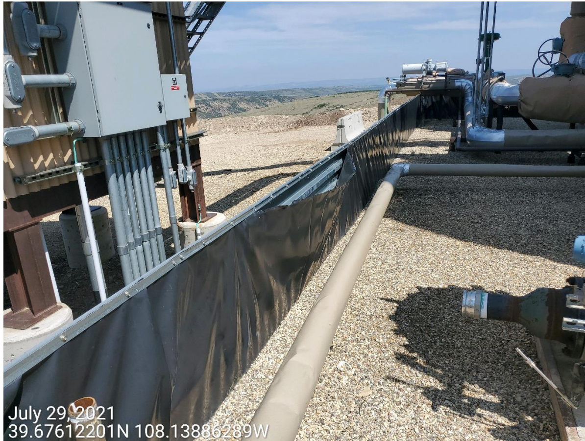
Photo 1: Photo taken from west end of the tank battery. Photo shows liner within secondary containment is in disrepair.
