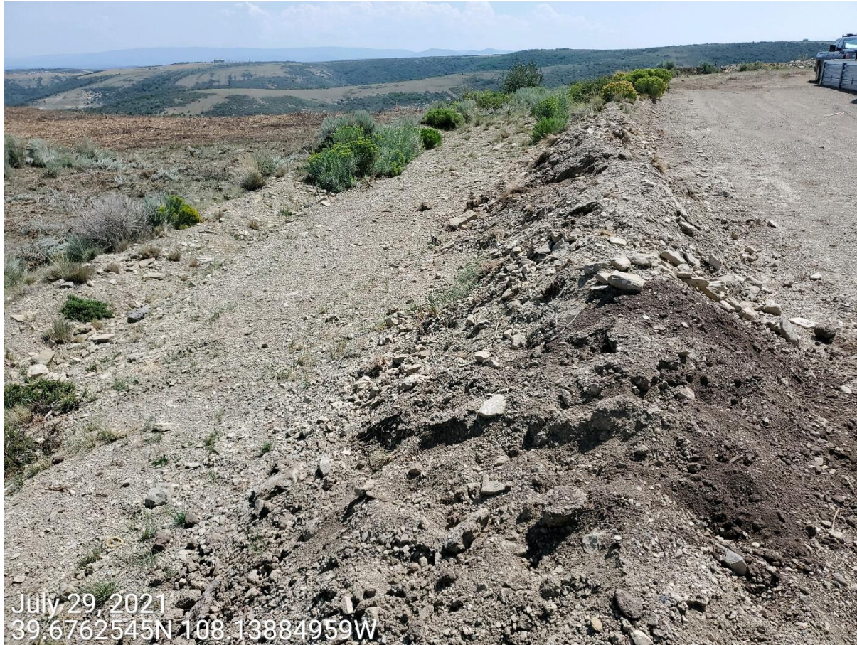
Photo 4: Photo taken from the north end of the Location, facing east. Photo shows slopes that remain loose material at risk to erosion; control measures to protect and stabilize slopes remain missing or insufficient.
