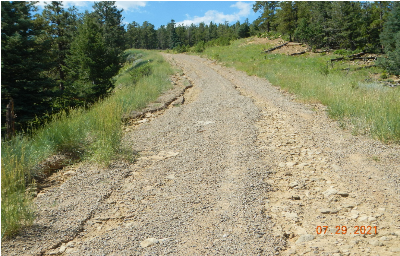
Photo 1. Facing southwest along the main road at Lat/Long:37.12487,-104.95788. There is erosion occurring down the road. Stormwater needs to be diverted off the road to prevent further erosion.
