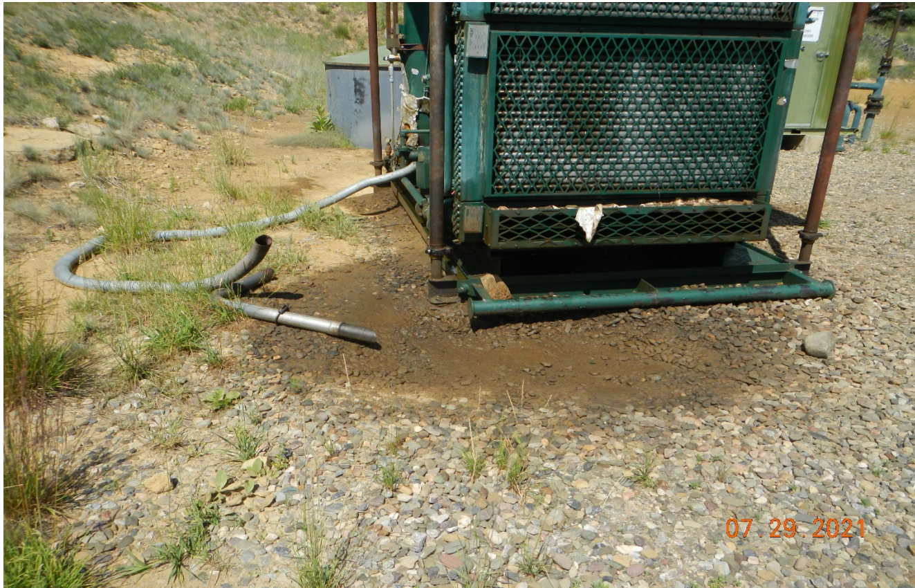
Photo 4. There is oil stained soils near the engine skid and oil inside the skid.
