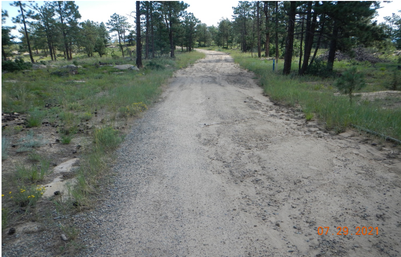
Photo 2. Facing northeast along the main road at Lat/Long:37.119485,-104.95374. There is erosion occurring down the road. Stormwater needs to be diverted off the road to prevent further erosion.
