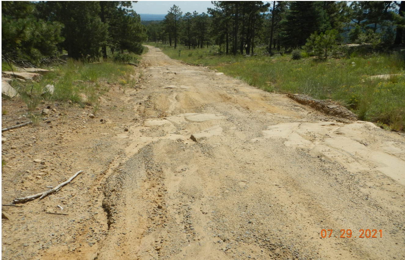
Photo 5. Traveling east along the main road near the location. This area has washed out and needs to be repaired.
