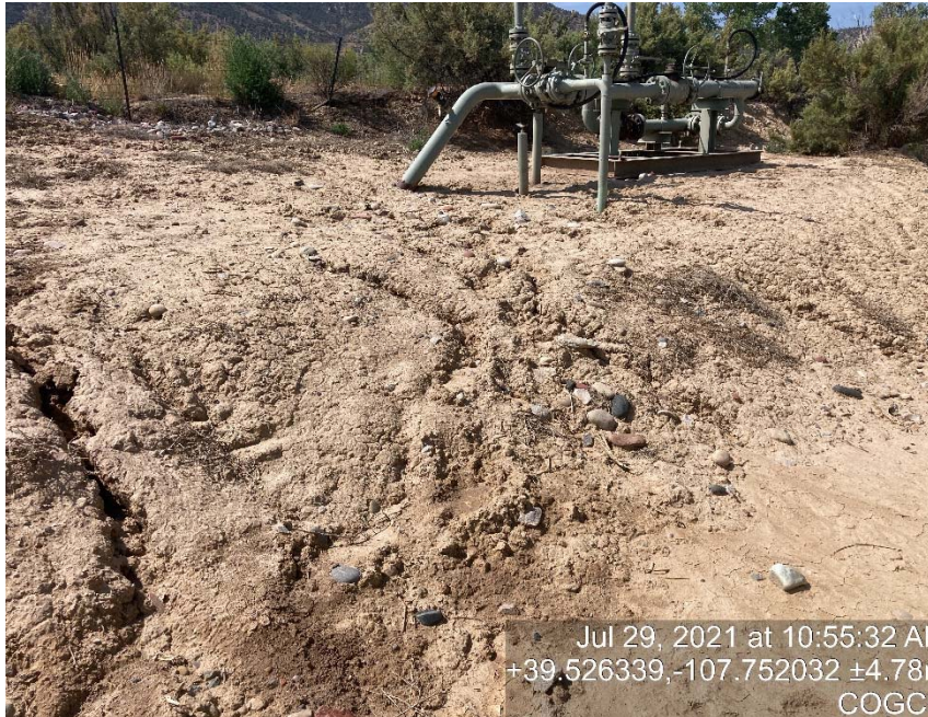
Lack of stabilization/erosion
