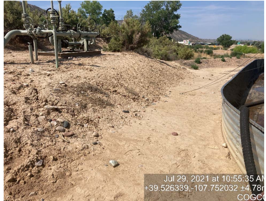
Lack of stabilization/erosion
