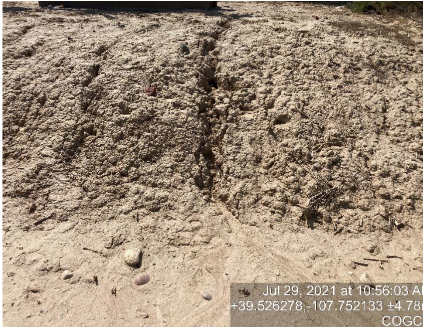
Lack of stabilization/erosion
