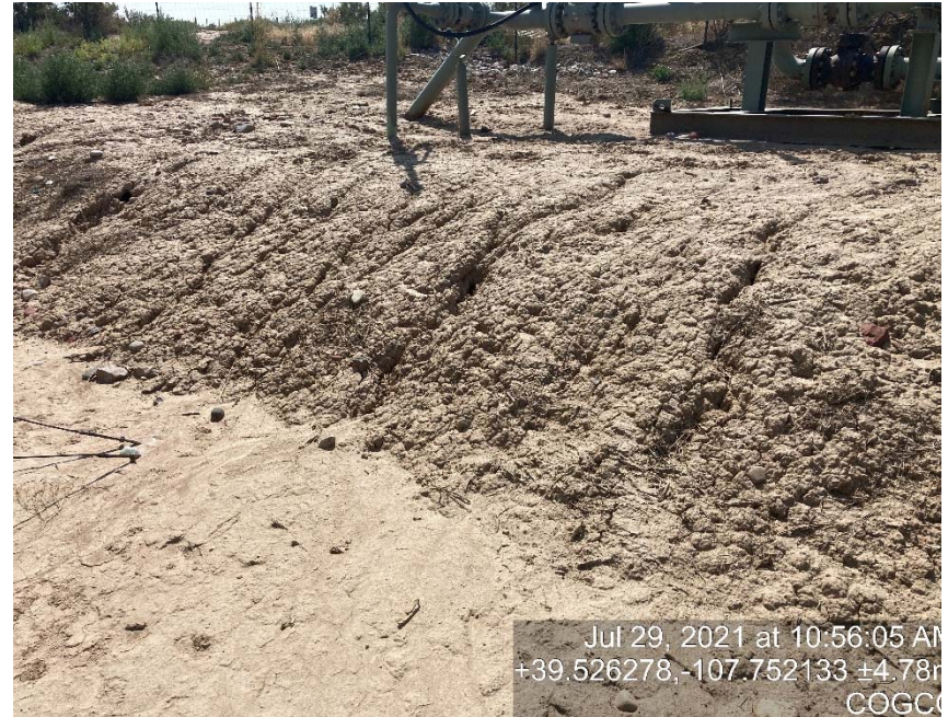
Lack of stabilization/erosion
