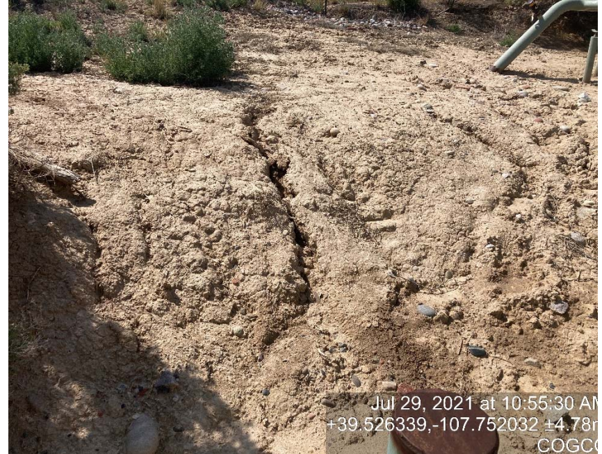
Lack of stabilization/erosion
