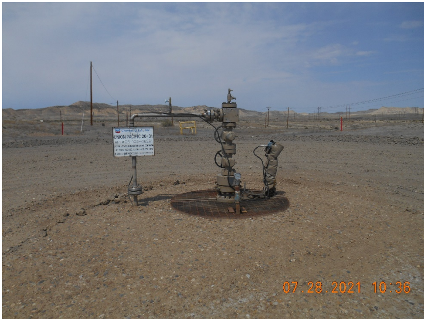
Injection wellhead
