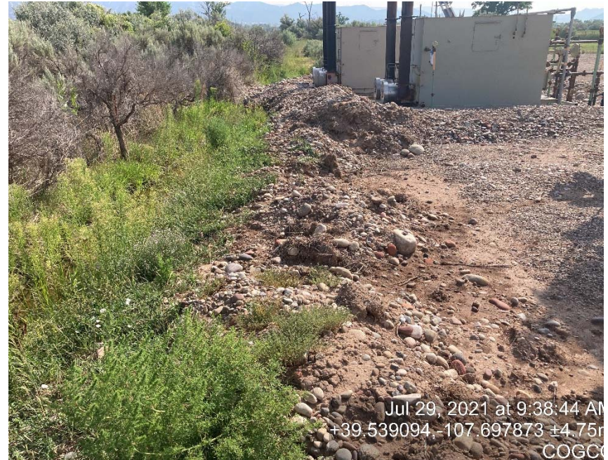
Loose soil pushed next to running ditch
