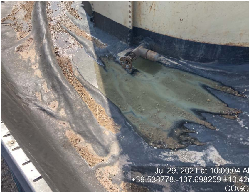
Drain valve actively leaking
