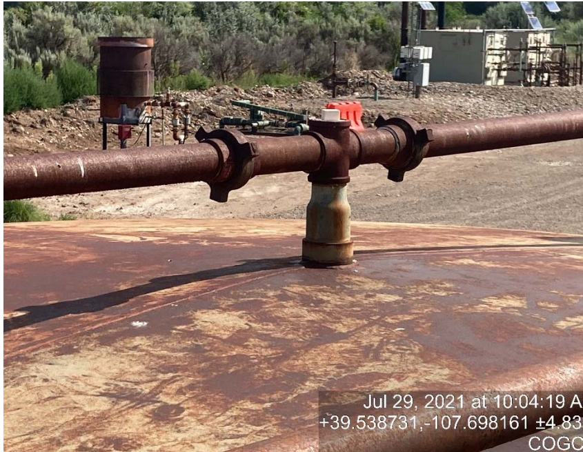
Plastic caps on top of tanks
