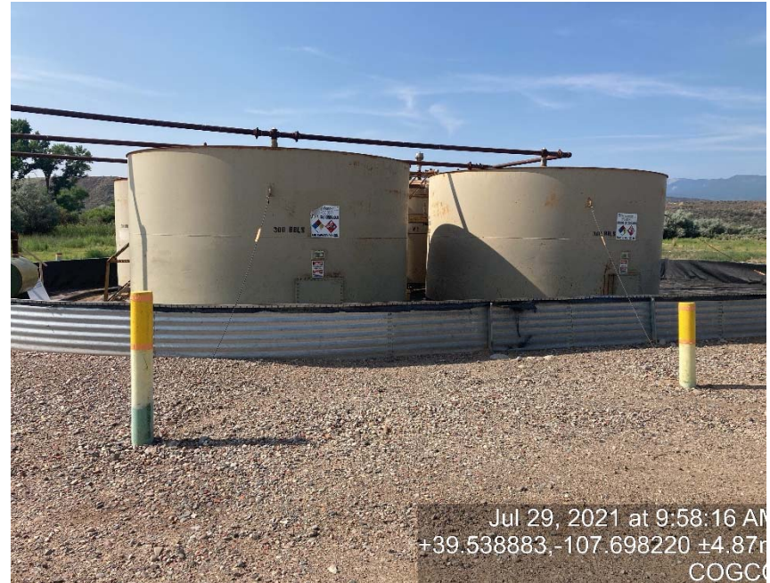
Location/Battery signage is not in a conspicuous location at tank battery
