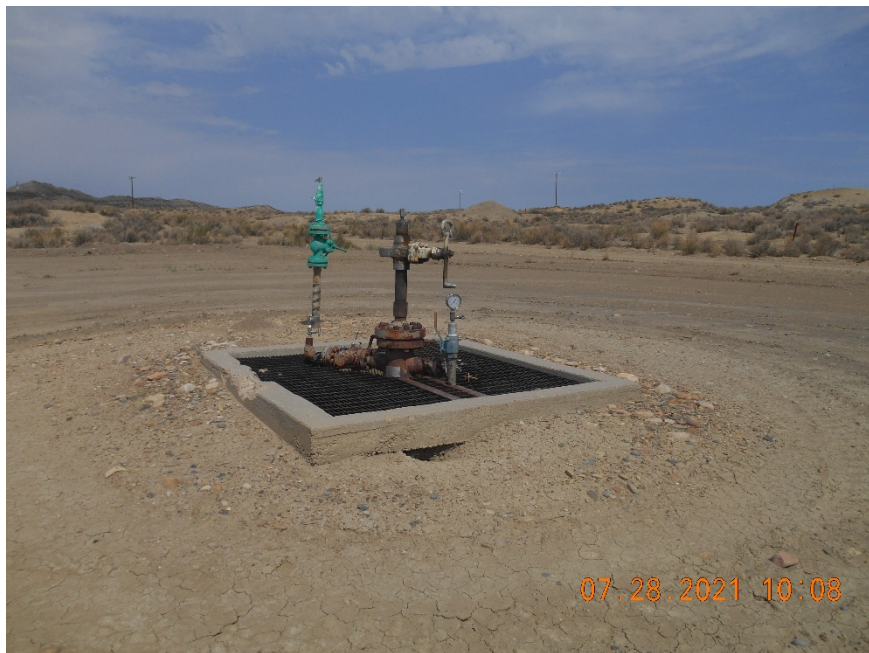
Injection wellhead. Temporarily Abandoned
