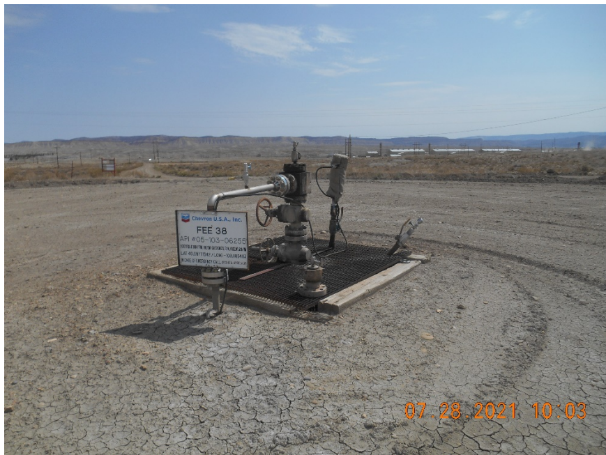
Injection wellhead.
