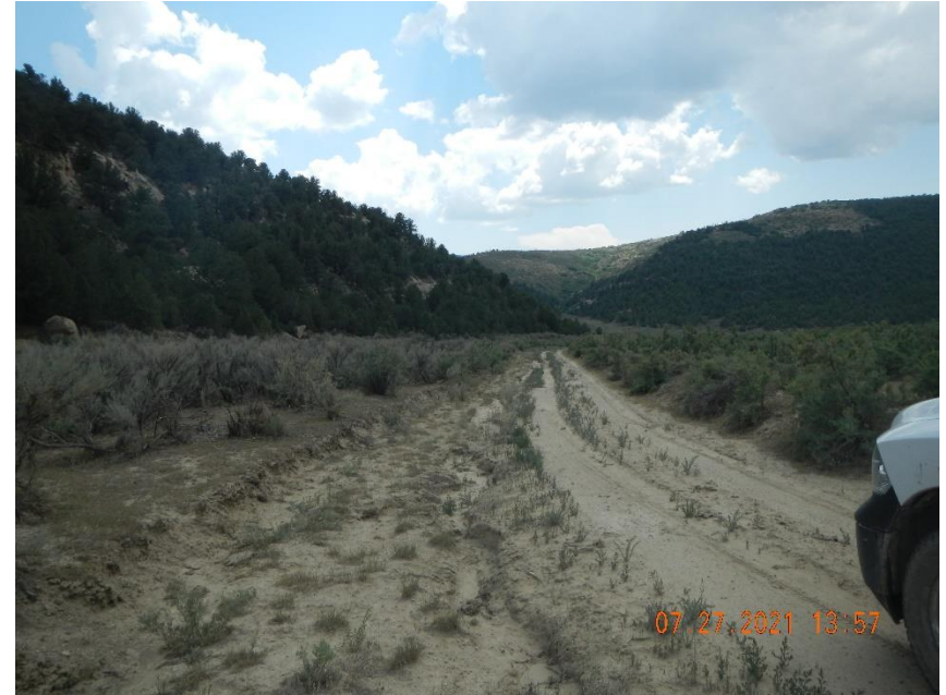
Road and storm water ditch not being maintained.
