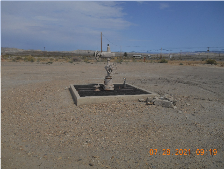
Injection wellhead. Temporarily Abandoned
