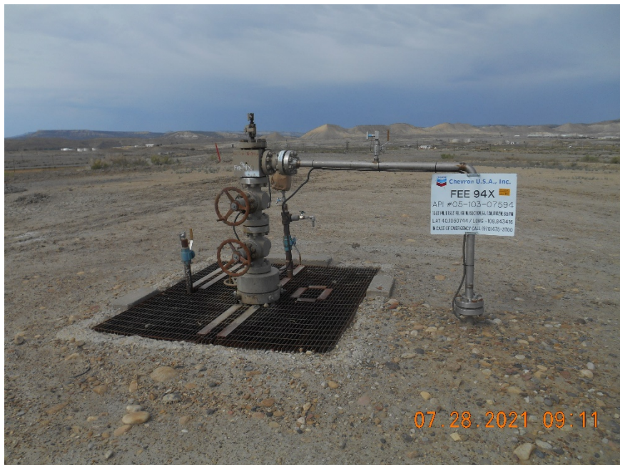
Injection wellhead
