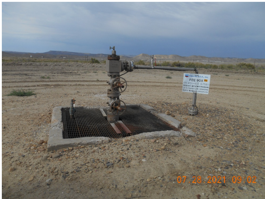
Injection wellhead
