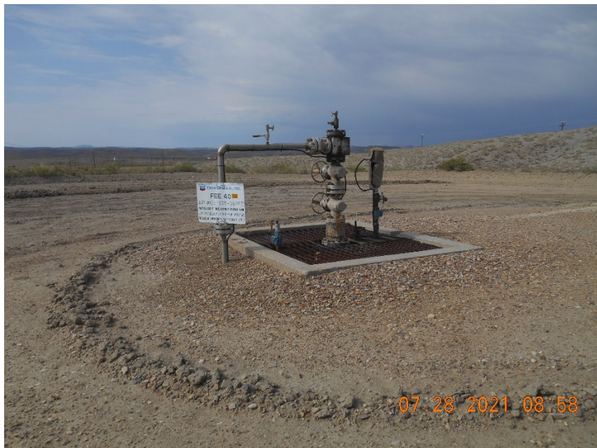
Injection wellhead
