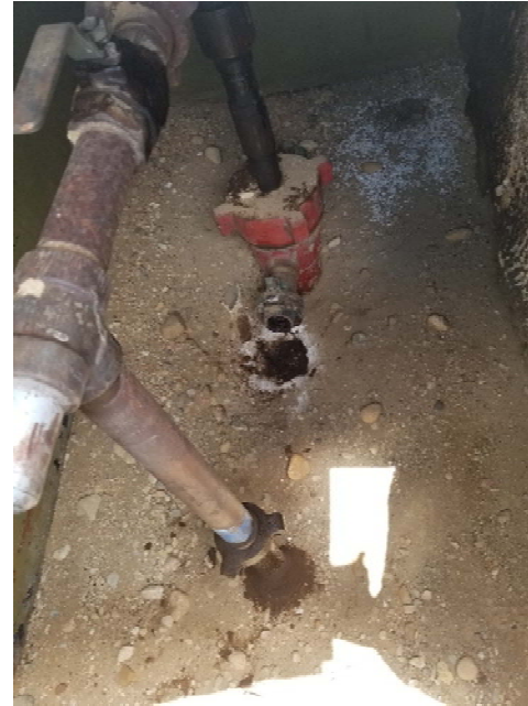
Photo 2. No bradenhead access apparent. Stained soil at wellhead.
