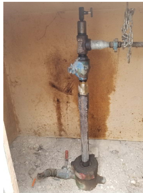
Photo 2. No bradenhead access apparent.
