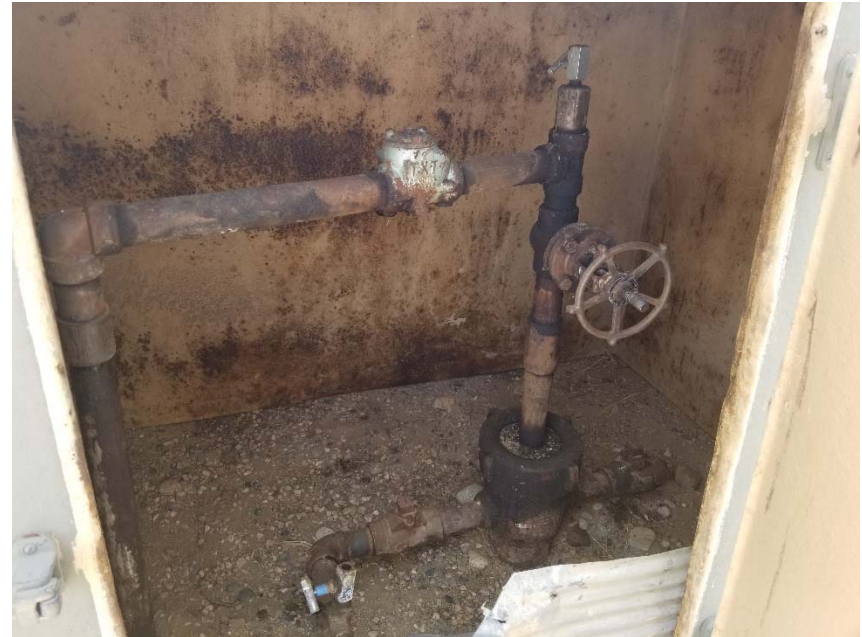
Photo 2. No bradenhead access apparent.
