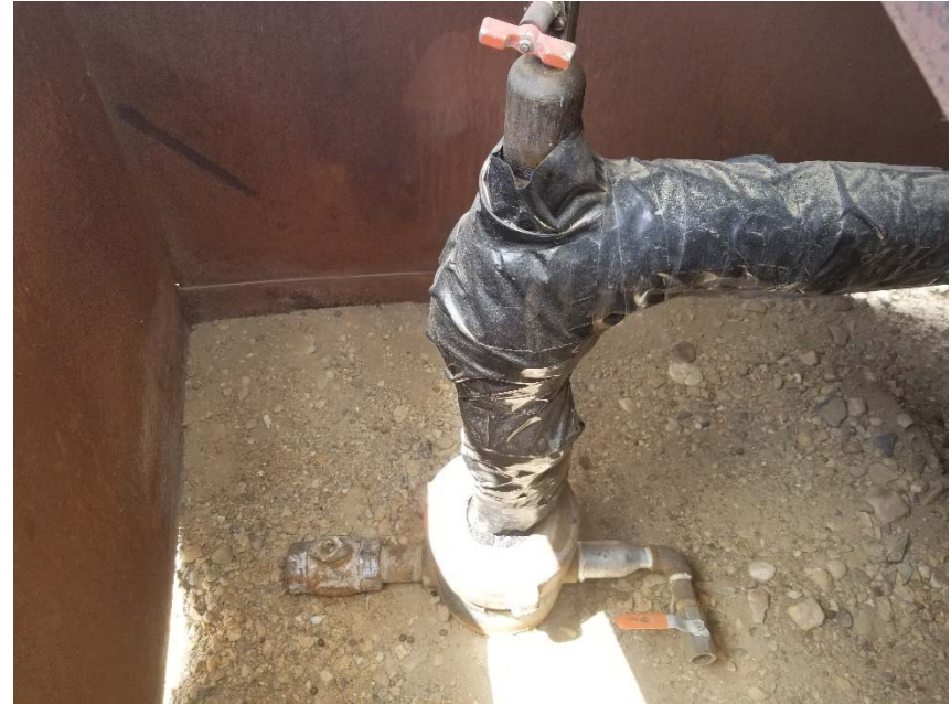
Photo 2. No bradenhead access apparent.
