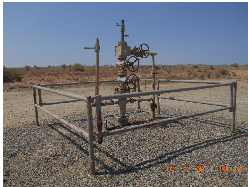
Wellhead Temporarily Abandoned
