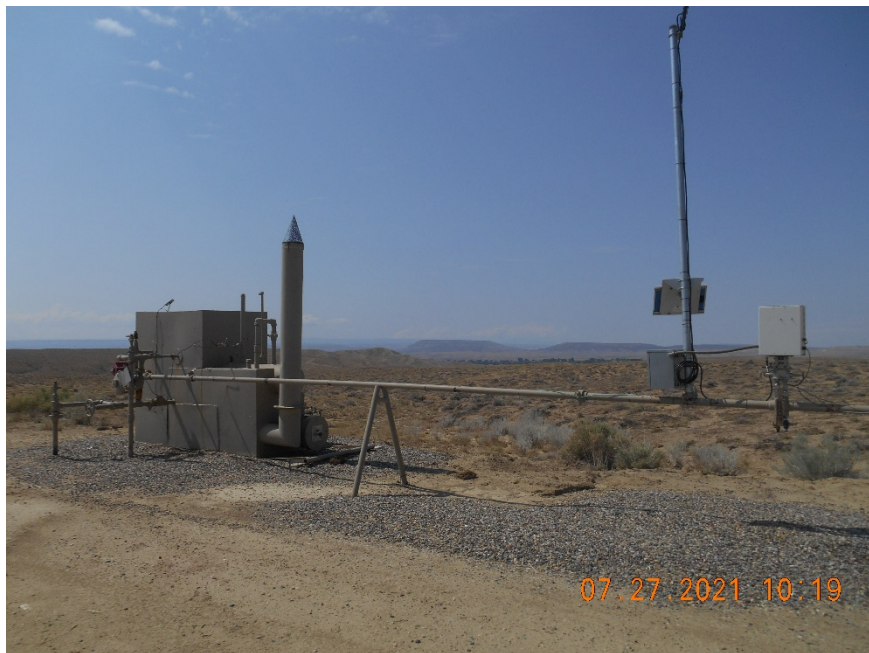
Separator with meter
