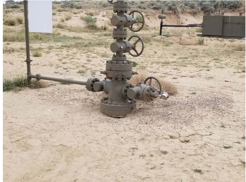
Photo 3. No bradenhead access apparent.
