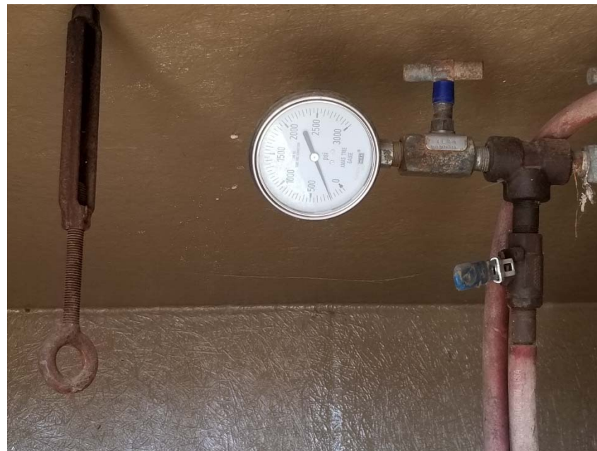
Photo 3. 200 psi on injection tubing.
