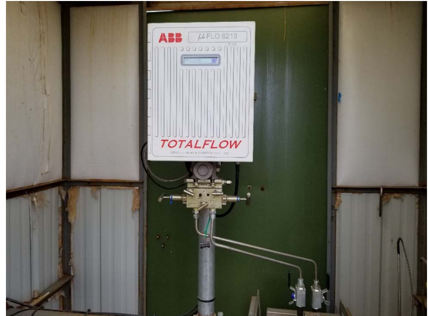
Photo 3. Gas meter not calibrated/calibration not displayed.
