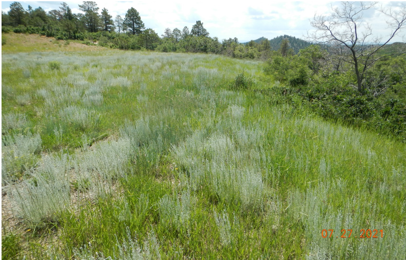
Photo 5. Facing southeast along the fill slope which is stabilized with vegetation cover.
