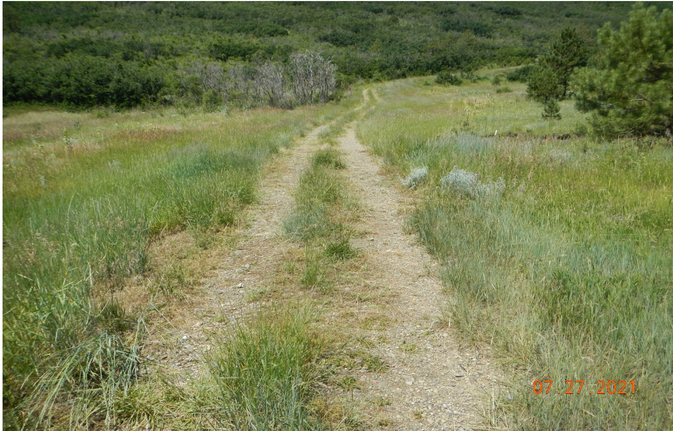
Photo 2. Facing southwest along the access road. The access road is stabilized with vegetation and gravel.
