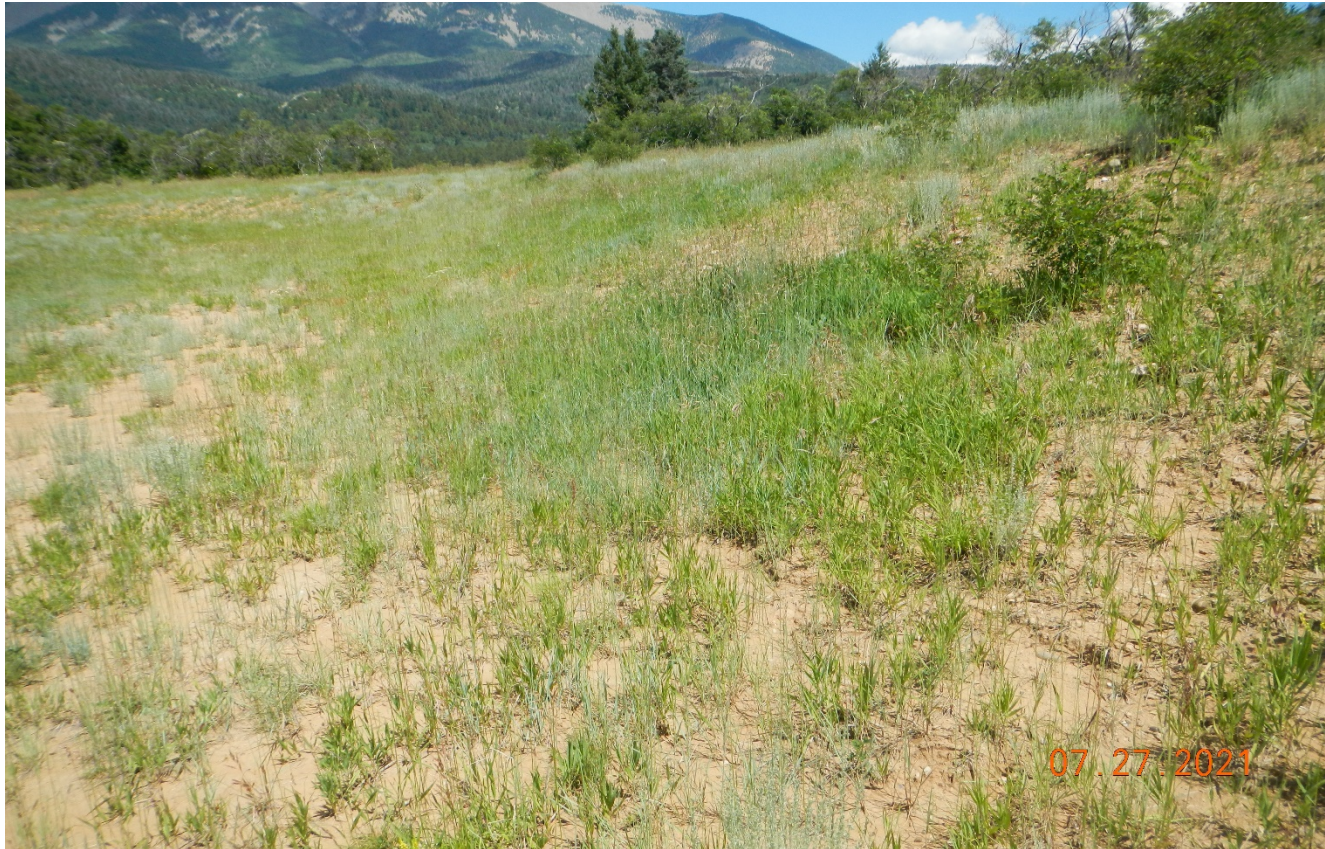
Photo 7. Facing northeast along the cut slope which is stabilized with vegetation cover.
