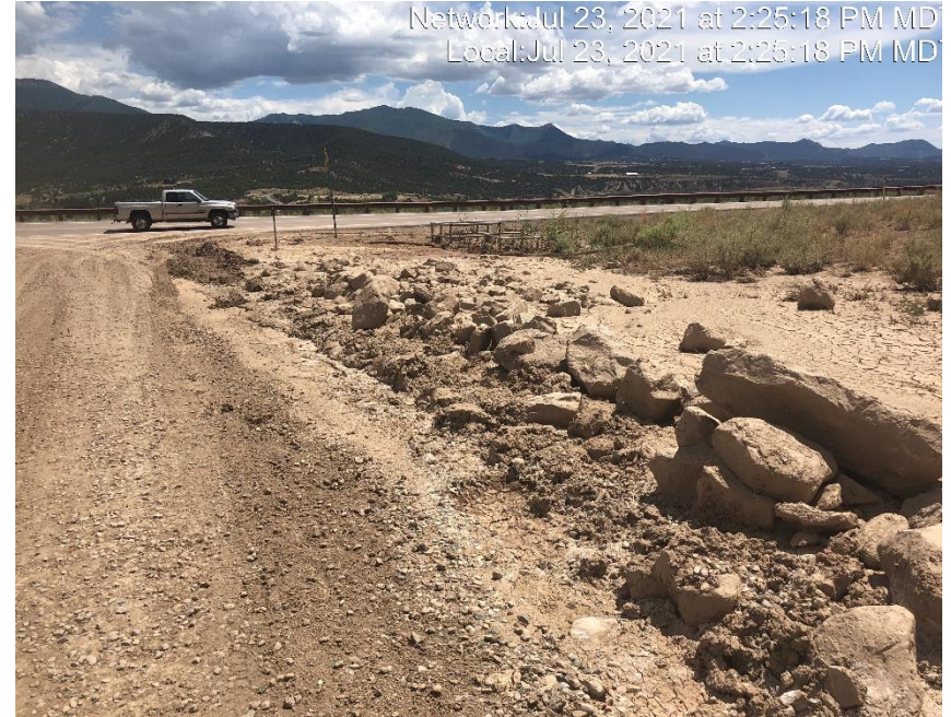
Photo #4598 Sediment and debris that was transported on to HWY 6.
