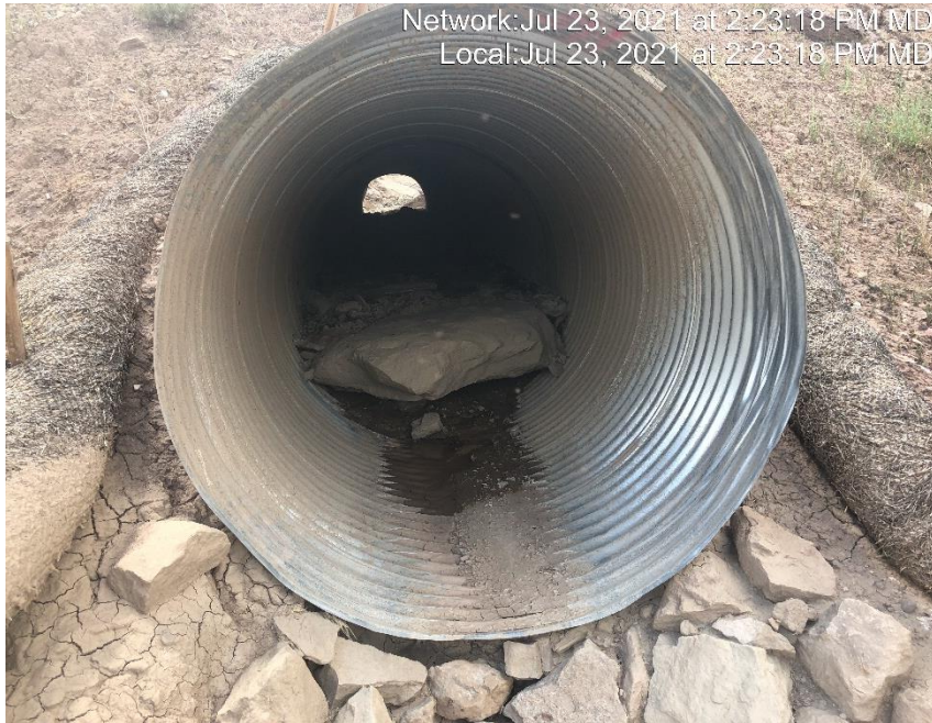
Photo #4595 Culvert capacity reduced do to sediment and debris.
