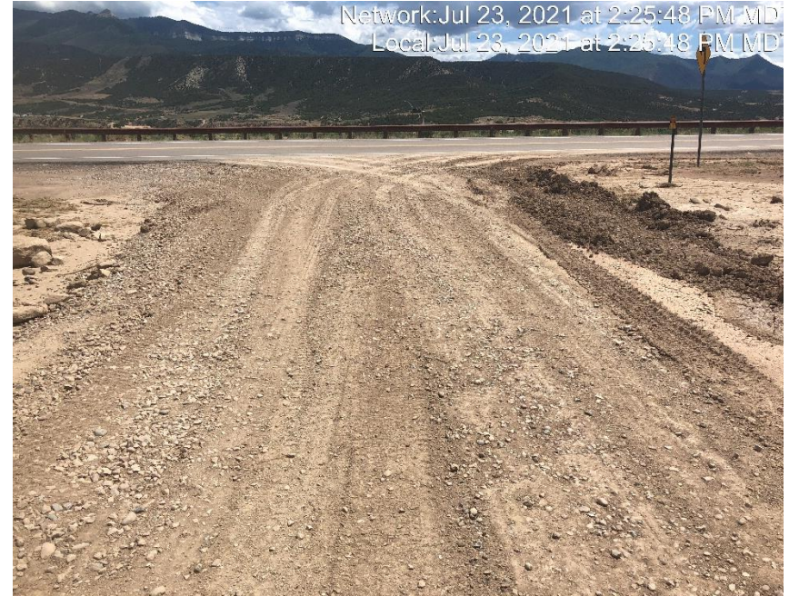
Photo #4600 Tracking BMP has not been implemented.
