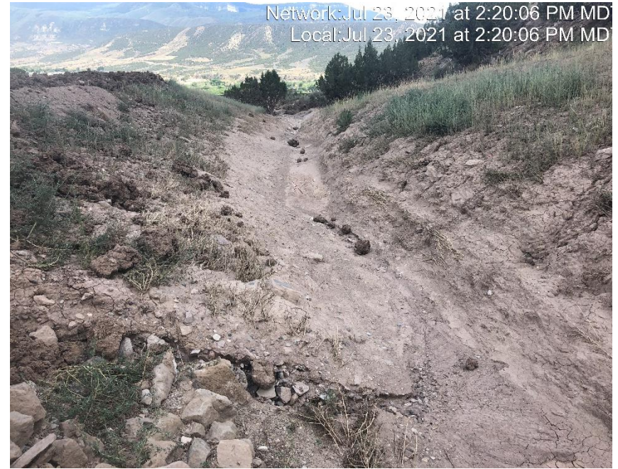
Photo #4592 Sediment has been bladed into ditch.
