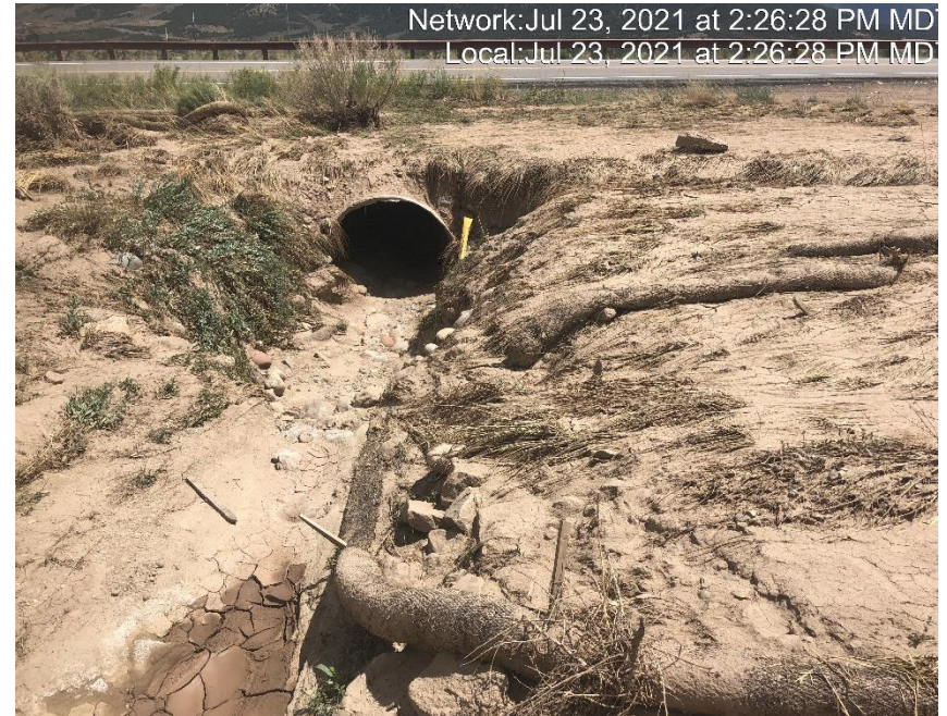
Photo #4602 Inlet of culver that runs under HWY 6.
