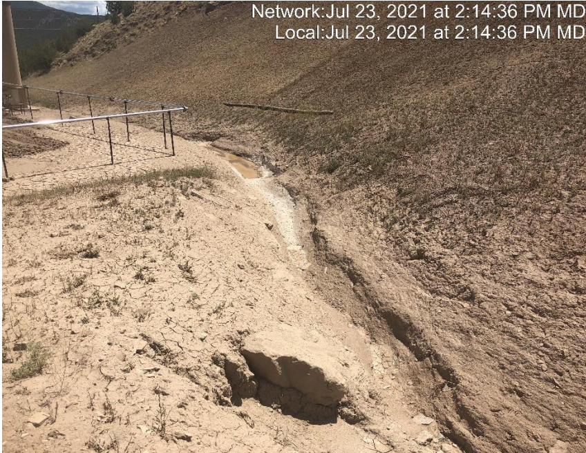
Photo #4585 Velocity checks have not been installed.
