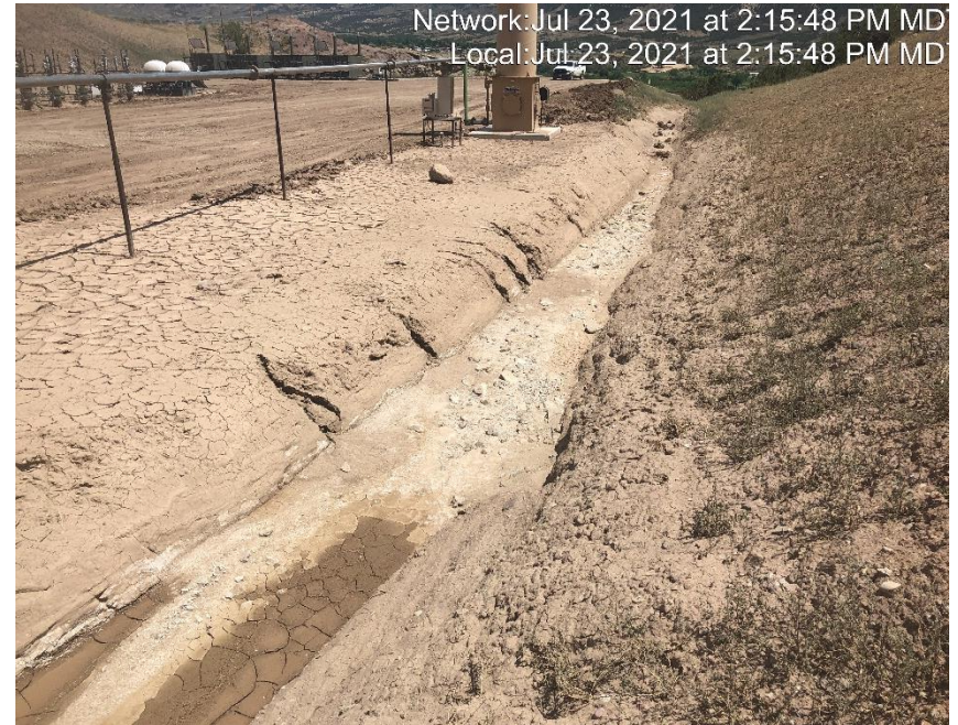
Photo #4587 Ditch shows signs of subsidence.
