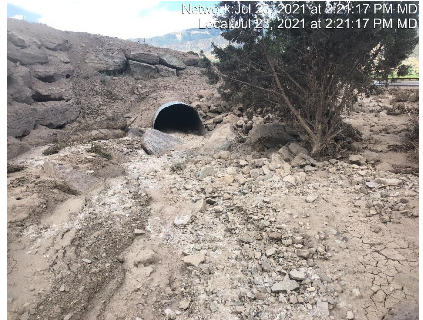
Photo #4593 Inlet of culvert under access road.
