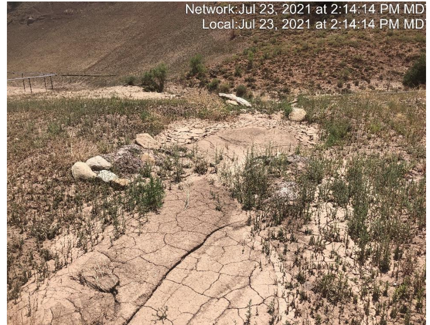
Photo #4584 Sediment trap filled with sediment.
