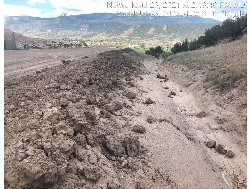
Photo #4589 Sediment has been bladed into ditch.
