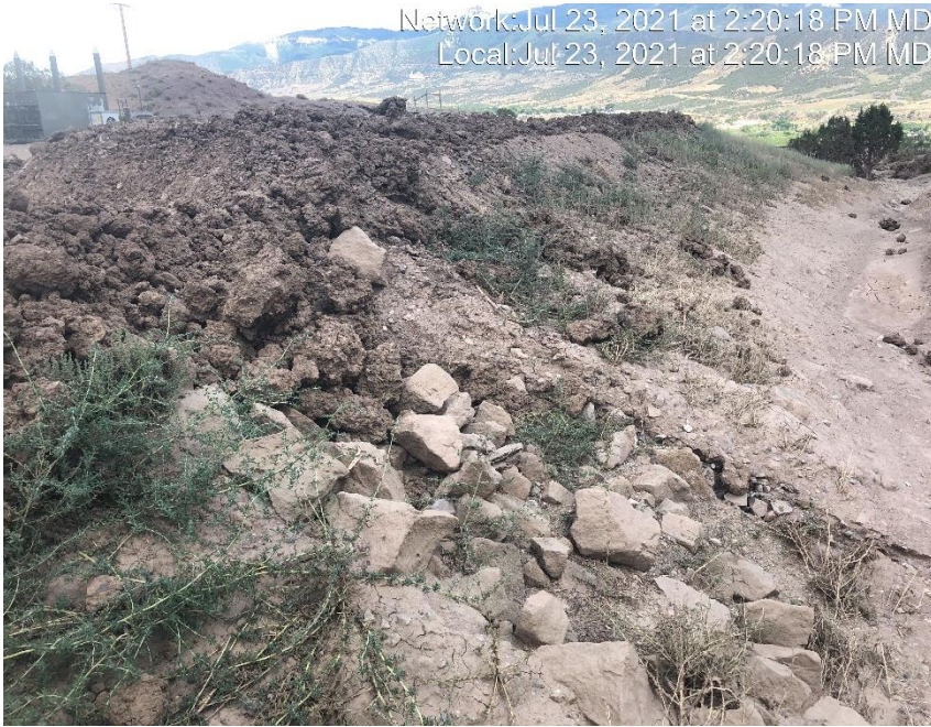
Photo #4591 Sediment has been bladed into BMP.
