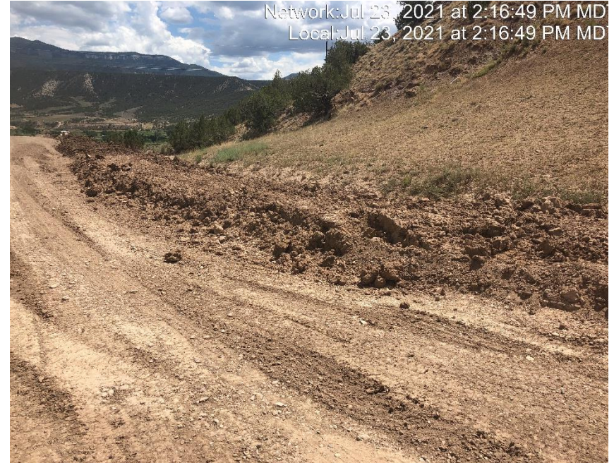
Photo #4588 Sediment has been bladed to the edge of ditch.
