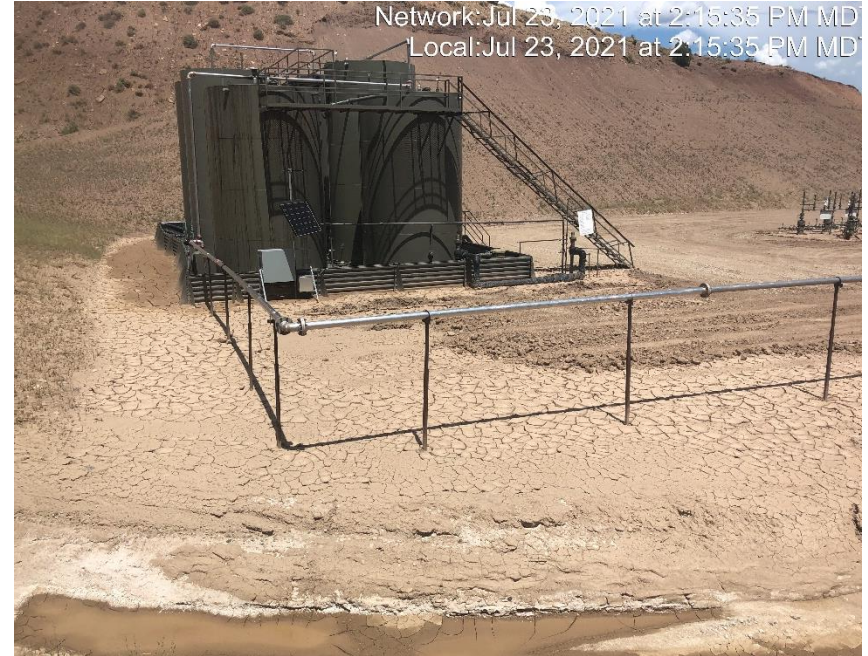
Photo #4586 Sediment encroaching on equipment.
