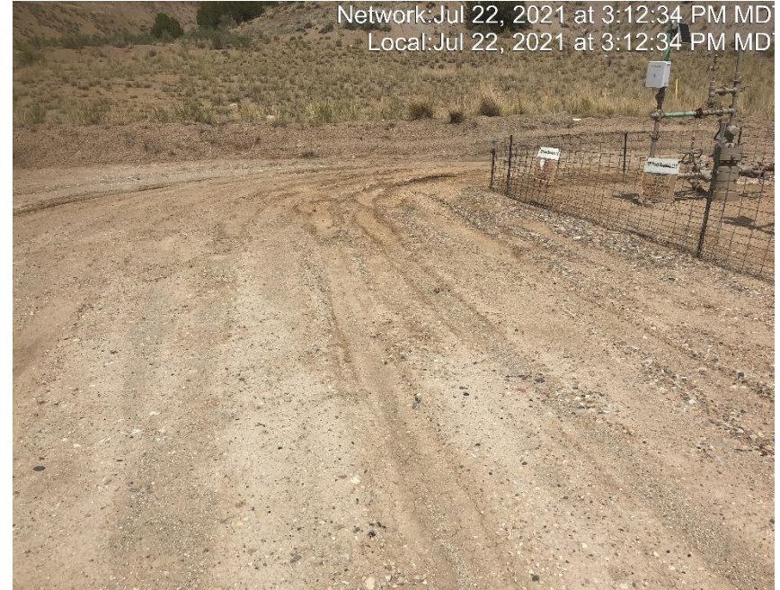
Photo #4568 Location lacks stabilization.
