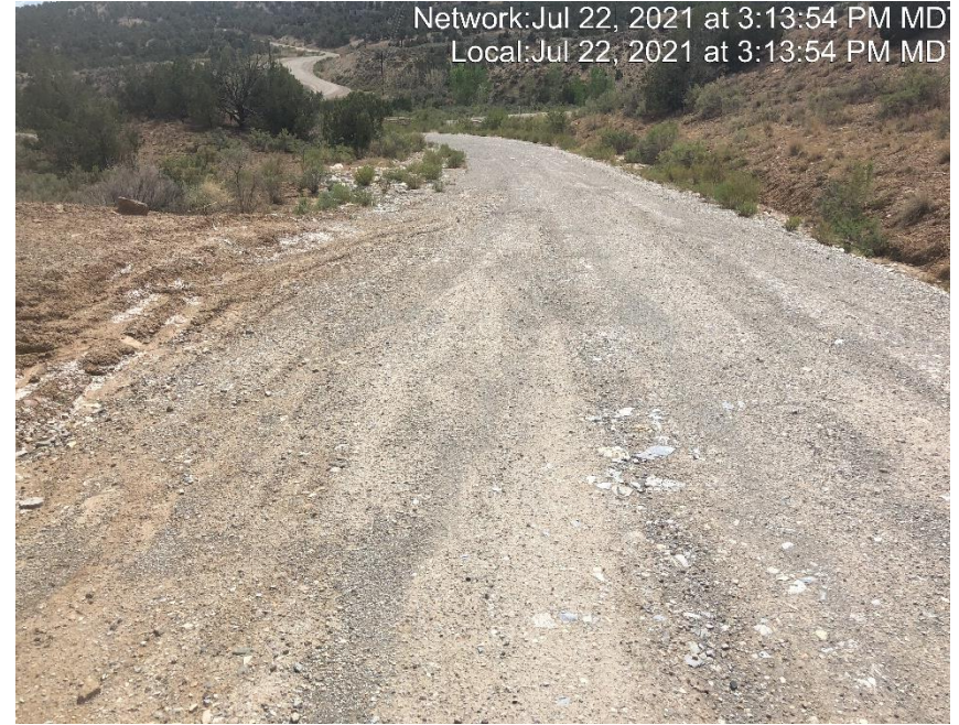
Photo #4772 No form of tracking BMP at entrance to location.
