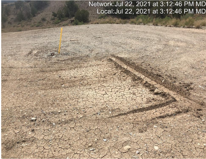
Photo #4569 Location lacks stabilization.
