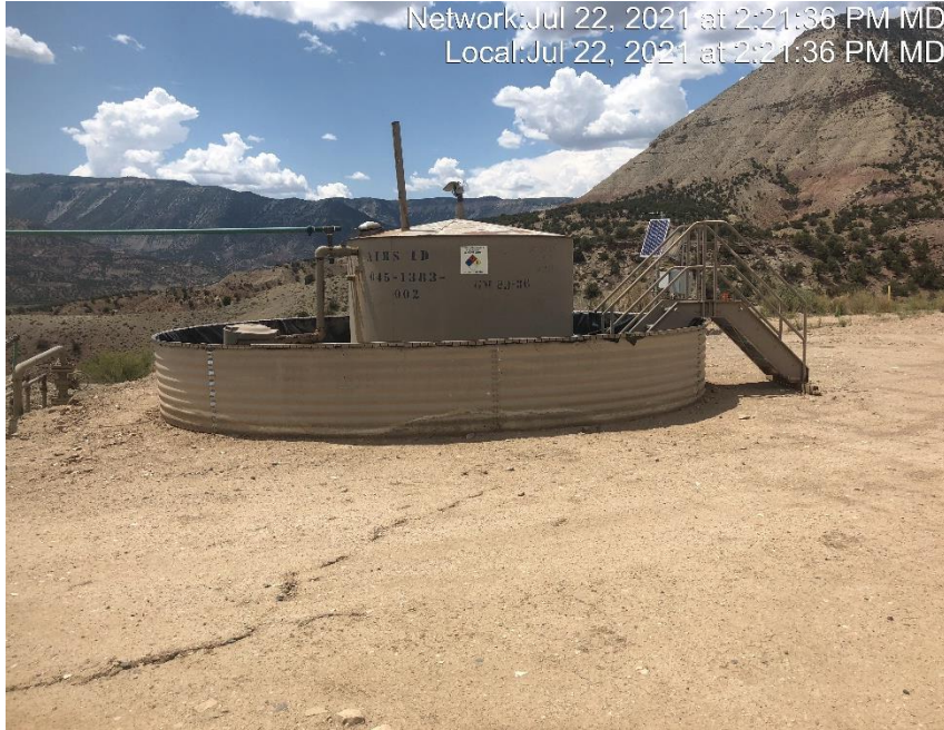
Photo #4559 No battery sign located at the tank battery.
