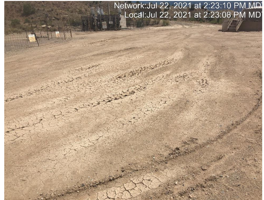
Photo #4561 Location lacks stabilization.
