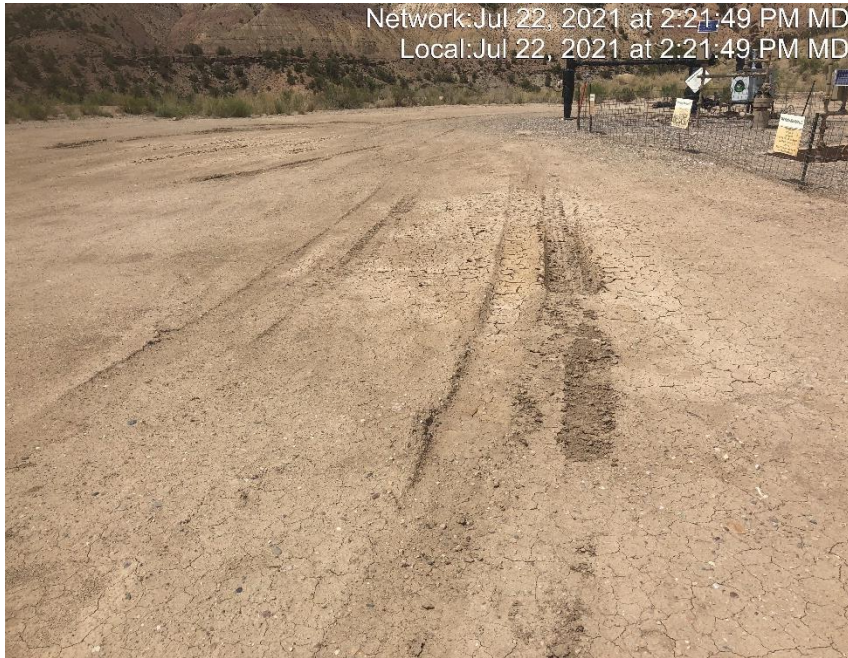
Photo #4560 Location lacks stabilization.
