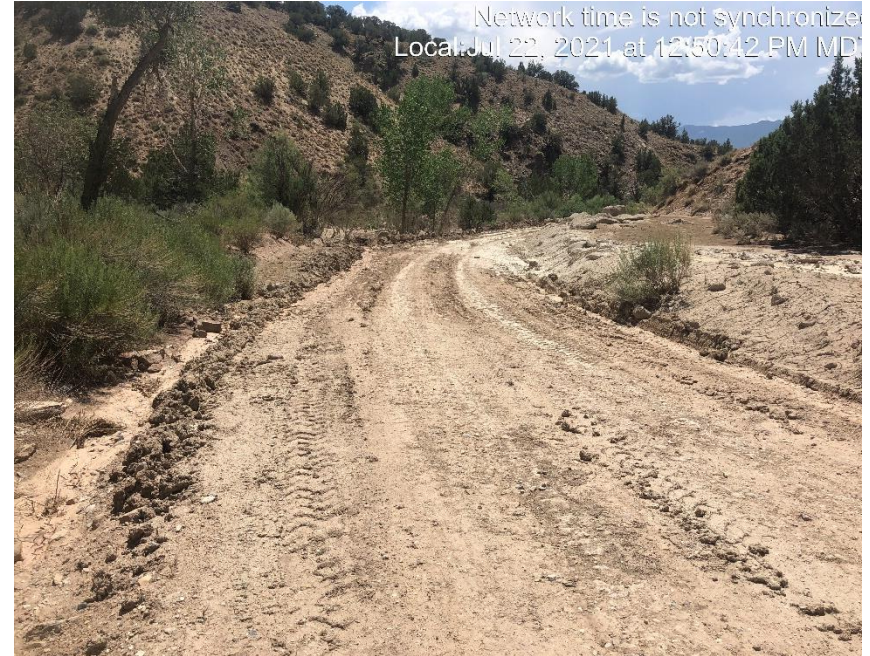
Photo #4540 Sediment and debris that over ran the access road.
