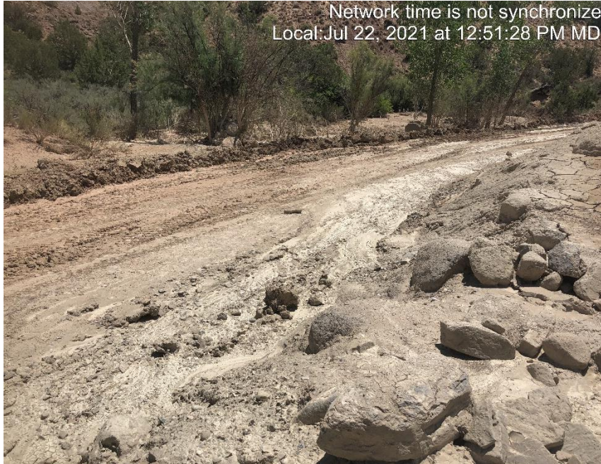
Photo #4543 Sediment and debris that over ran the access road.
