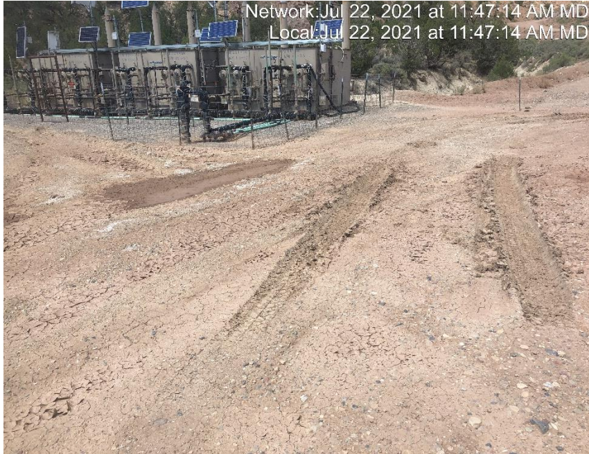
Photo #4537 Location lacks stabilization.
