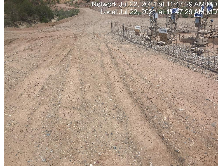
Photo #4538 Location lacks stabilization.
