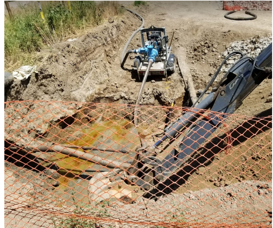
Photo 4 – Spill excavation being backfilled. Impacts remain visible in-situ and free product visible on groundwater.
