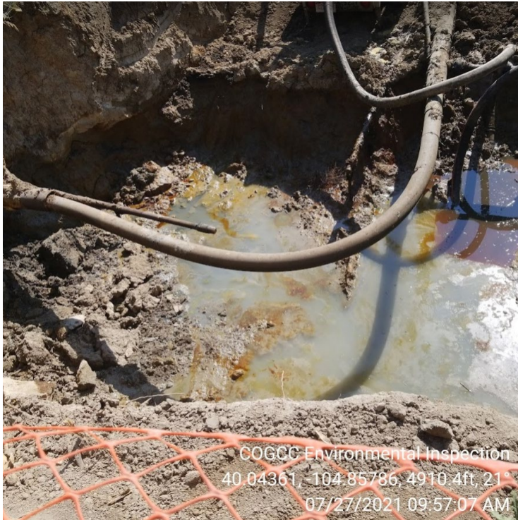
Photo 3 – Spill excavation. Impacts remain in situ. Free product visible on groundwater.
