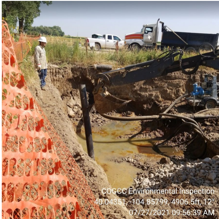
Photo 1 – Spill excavation. Impacts remain in situ. Free product visible on groundwater.
