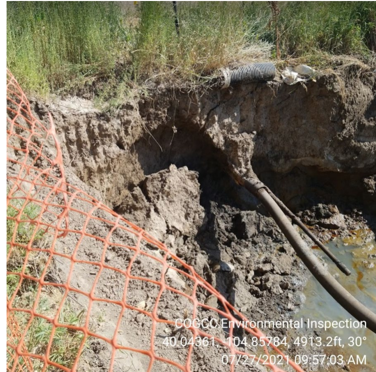
Photo 2 – Spill excavation. Impacts remain in situ. Free product visible on groundwater.
