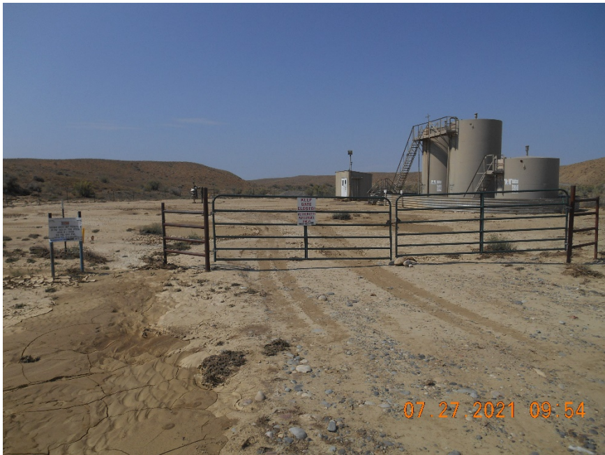
Location overview looking SW.
