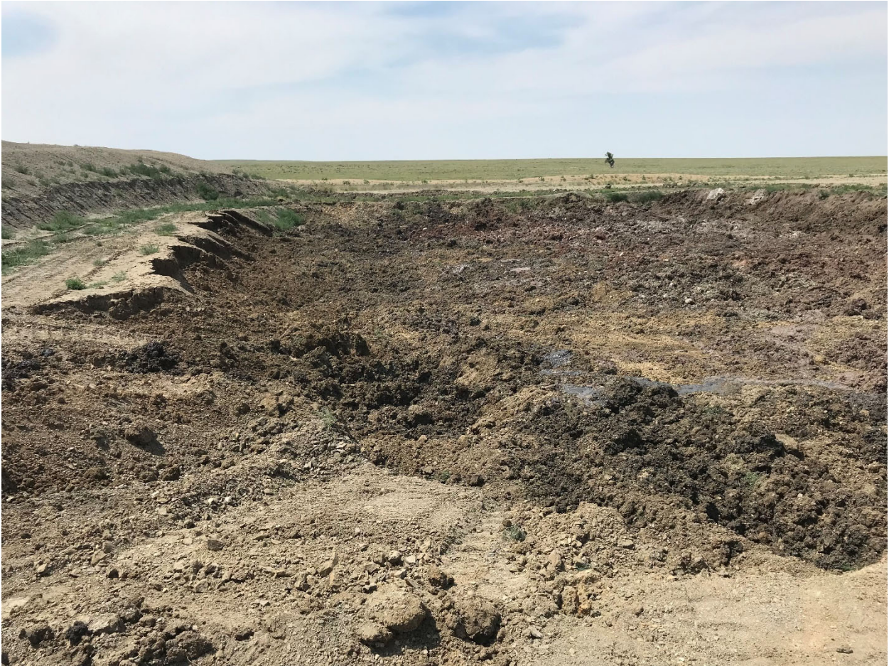
Pit after mixing facing northwest 6/18/21
