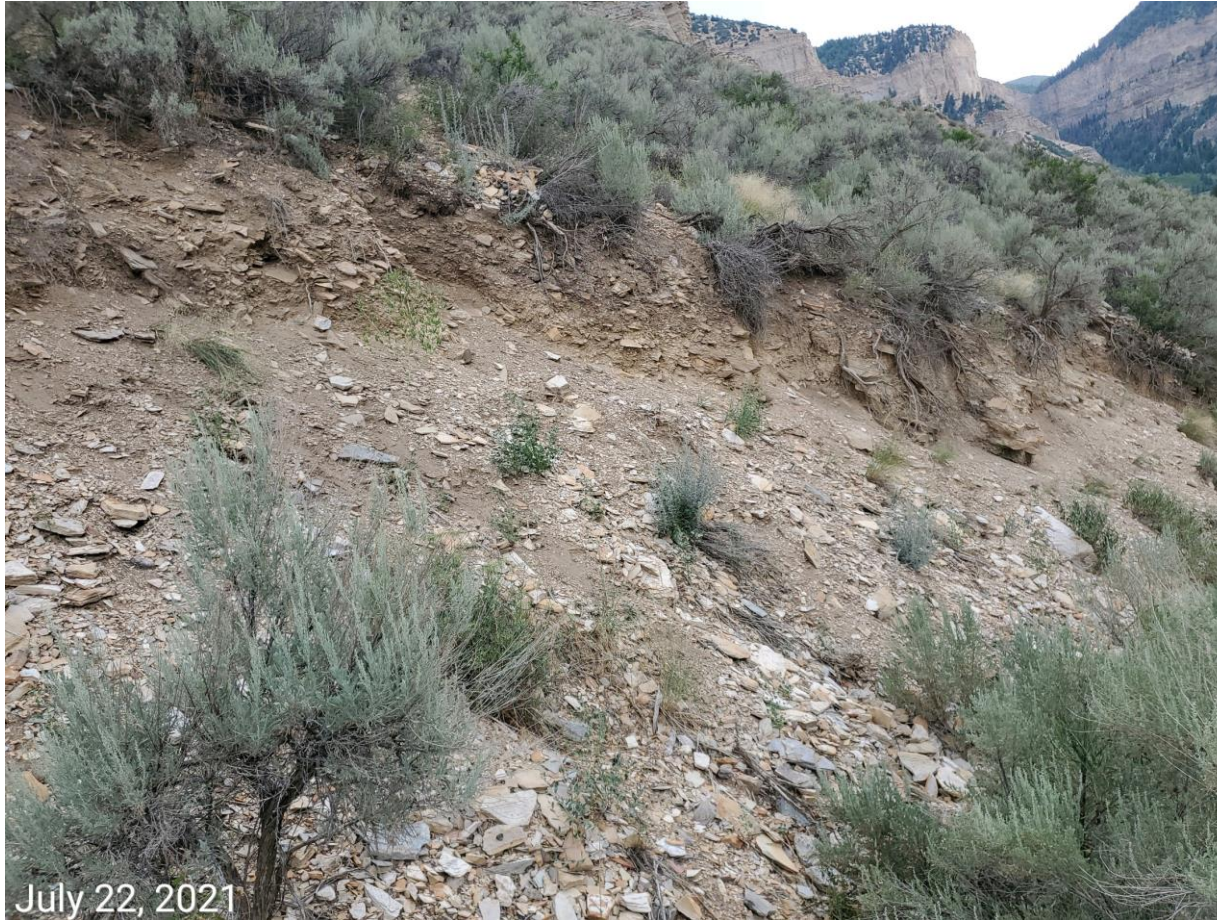
Photo 1: Photo taken from the diversion ditch along the north end of the Location, facing northeast. Photo shows example of areas within the ditch that are not stabilize resulting in erosion degradation offsite and up the slope. BMPs to protect and stabilize the slopes remain missing or insufficient.
