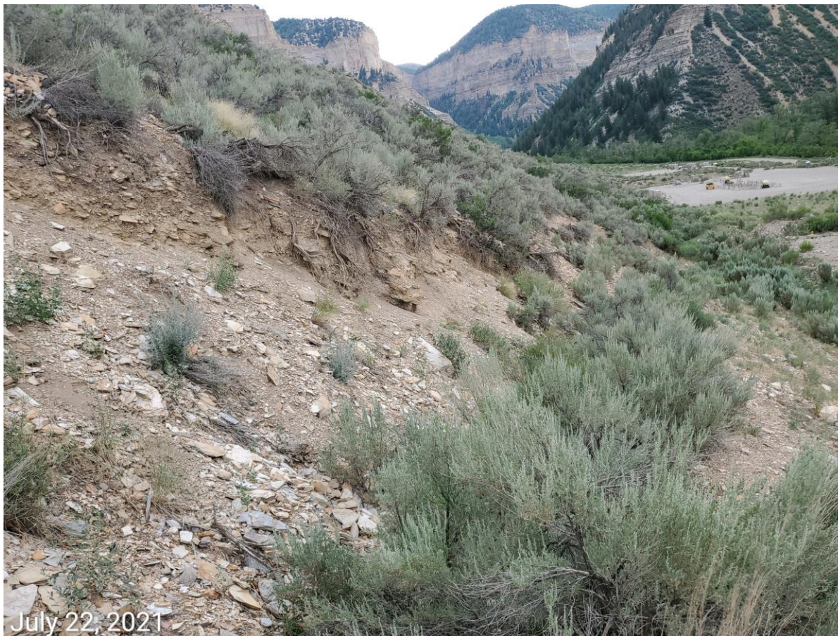
Photo 2: Photo taken from the diversion ditch along the north end of the Location, facing northeast. Photo shows example of areas within the ditch that are not stabilize resulting in erosion degradation offsite and up the slope. BMPs to protect and stabilize the slopes remain missing or insufficient.
