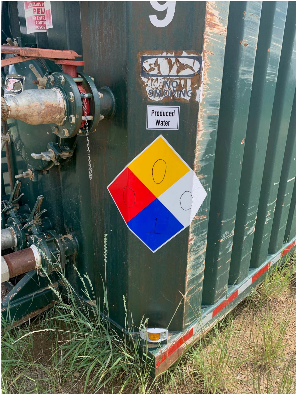
Applied labeling to tank to comply with Rule 605.h.(1).
