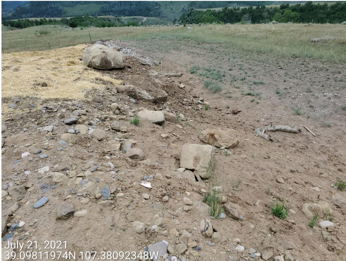
Photo 1: Photo taken from the west end of the Location, facing south. Photo shows control measures to protect and stabilize the slopes on the west end of the Location remain missing, or insufficient.
