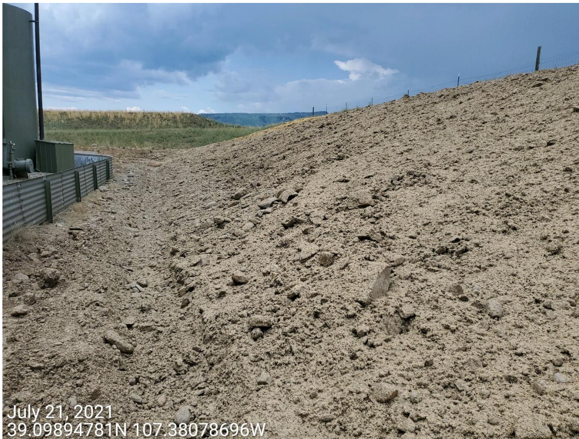
Photo 5: Photo taken from the cuts lopes on the north end of the Location, facing west. Photo shows slopes have been regraded, and a hydromulch applied to stabilize the soils. This portion of the CA has been addressed.
