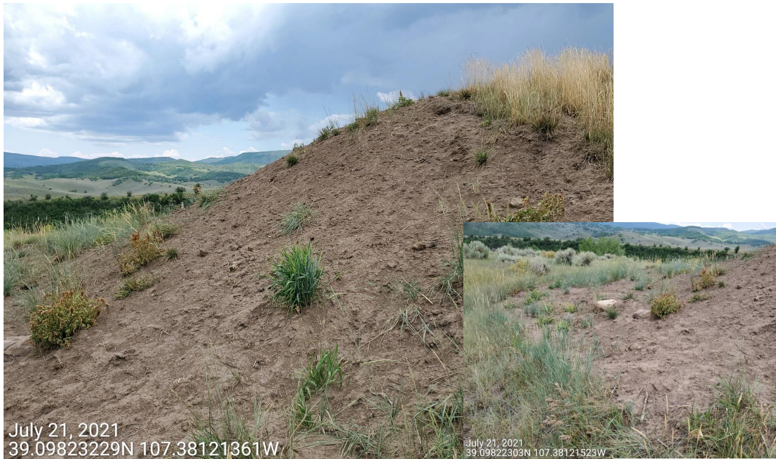
Photo 3: Photo taken from the topsoil stockpile on the northwest end of the Location. Photos show control measures to protect and stabilize the soils at the stockpile remain missing, or insufficient.
