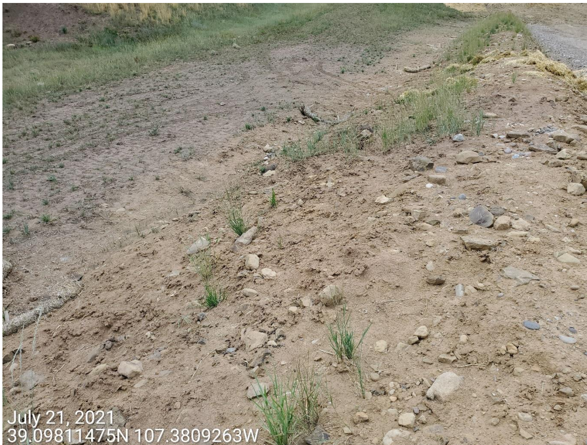
Photo 2: Photo taken from the west end of the Location, facing northwest. Photo shows control measures to protect and stabilize the slopes on the west end of the Location remain missing, or insufficient.
