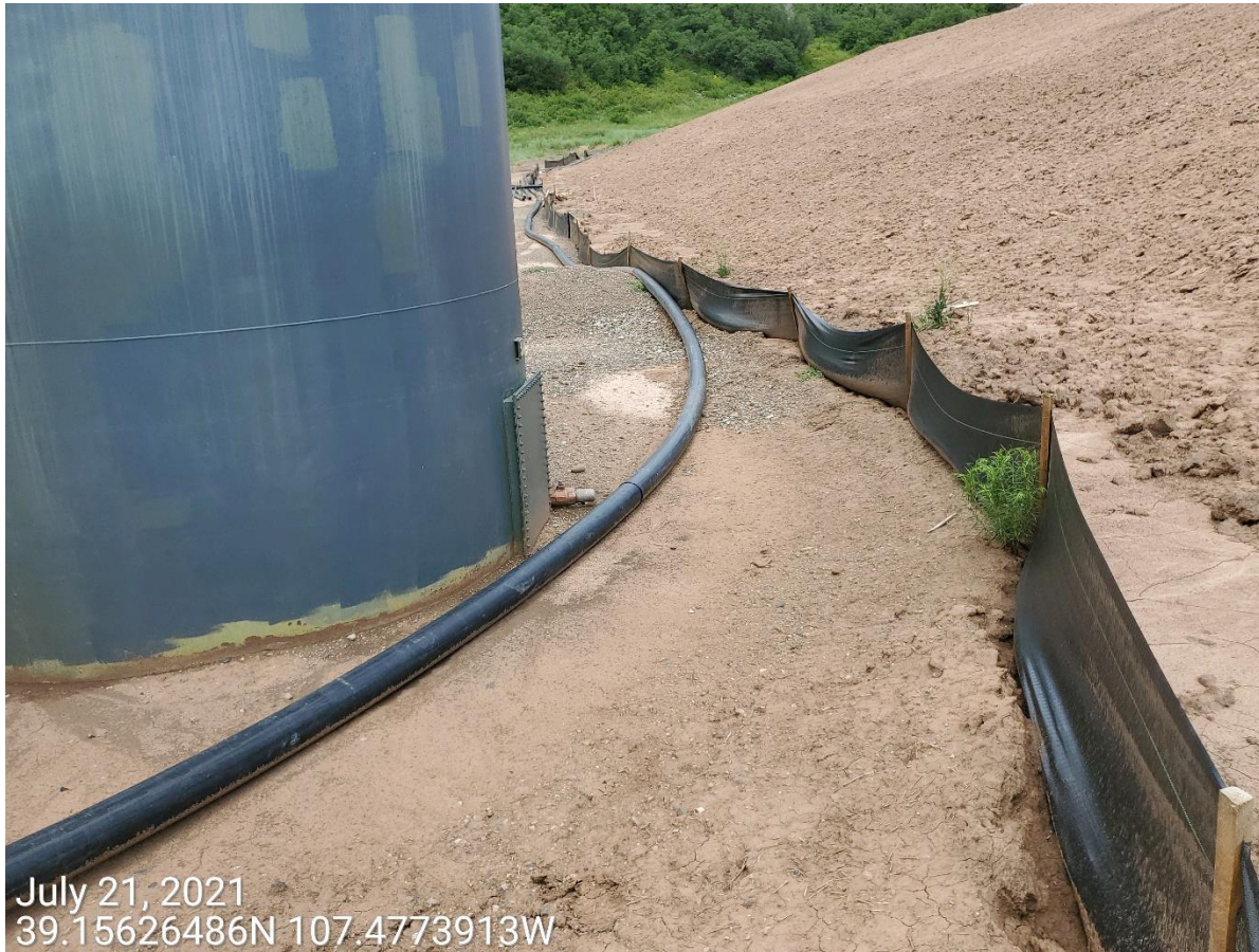
Photo 14: Photo shows secondary containment around the tank battery remains inadequate.
