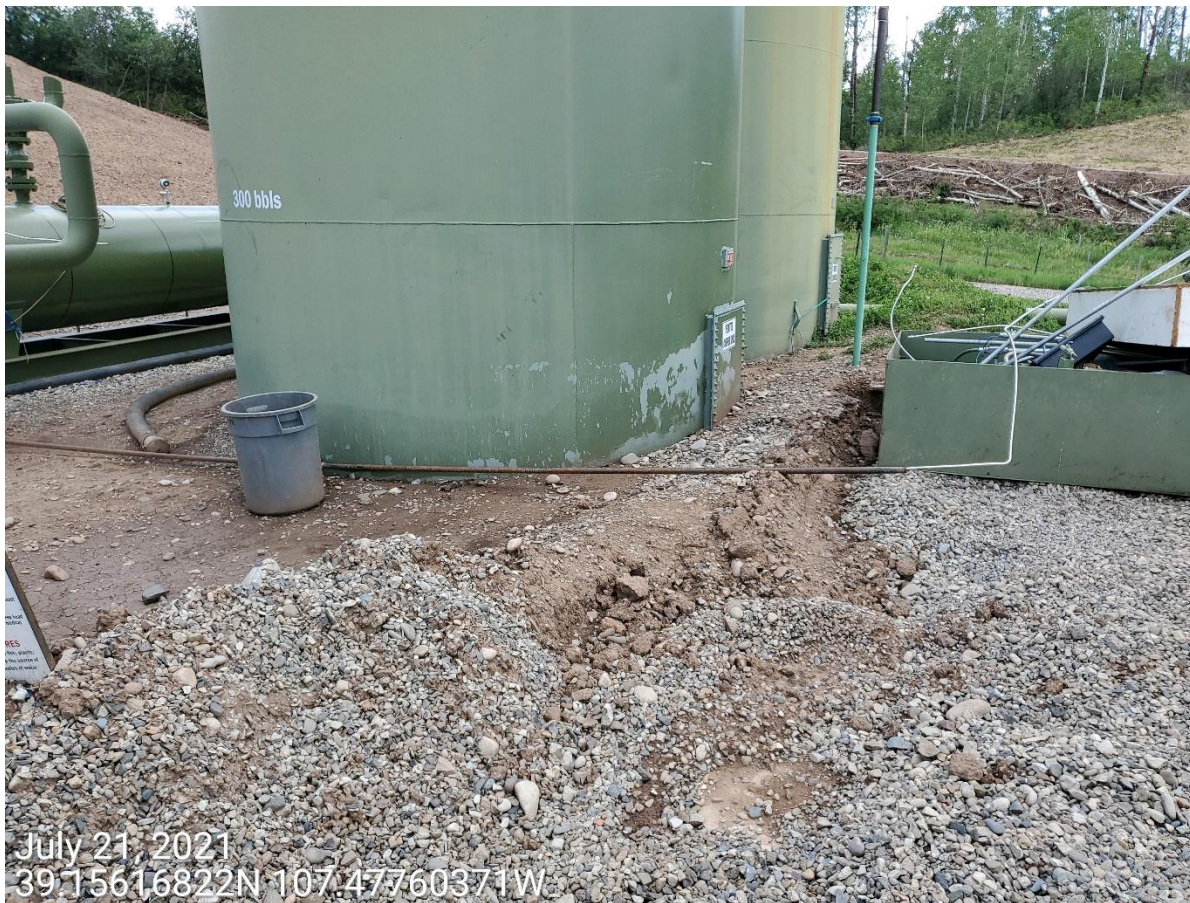
Photo 13: Photo shows secondary containment around the tank battery remains inadequate.
