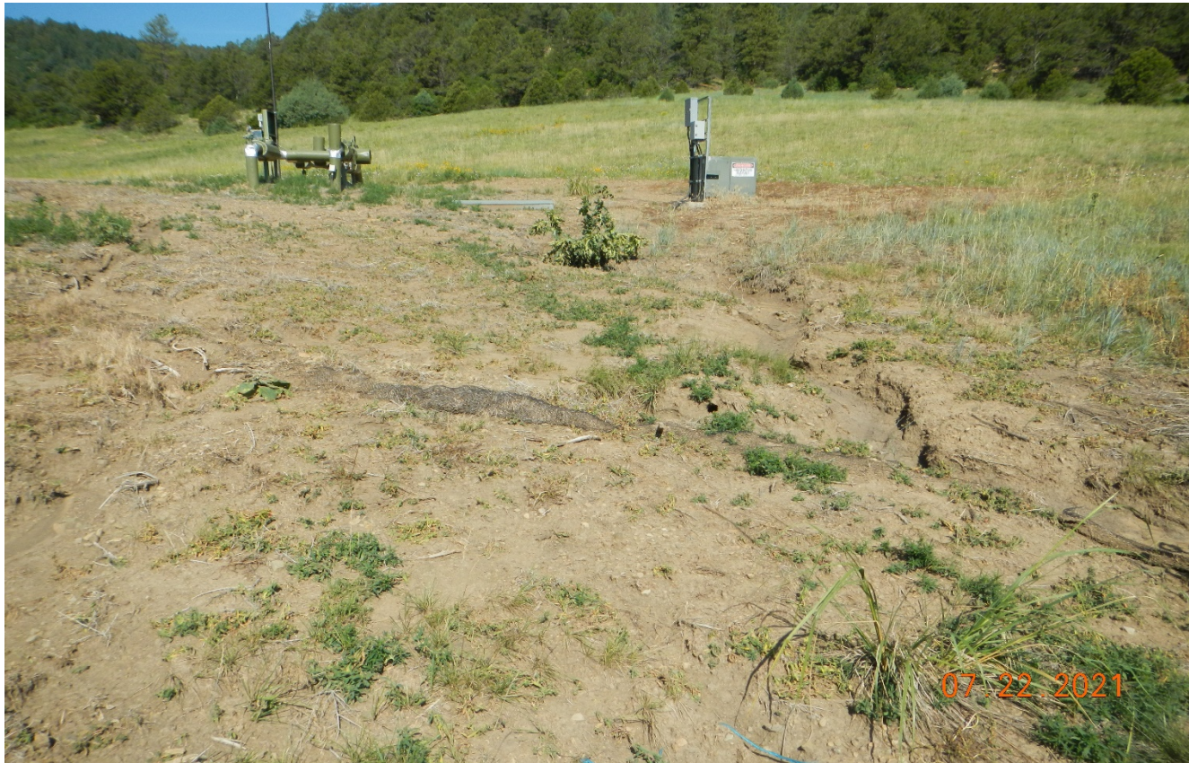
Photo 5. Facing west at the northeast side of the location. This area is not stabilized and there is an erosion channel that will need to be repaired.
