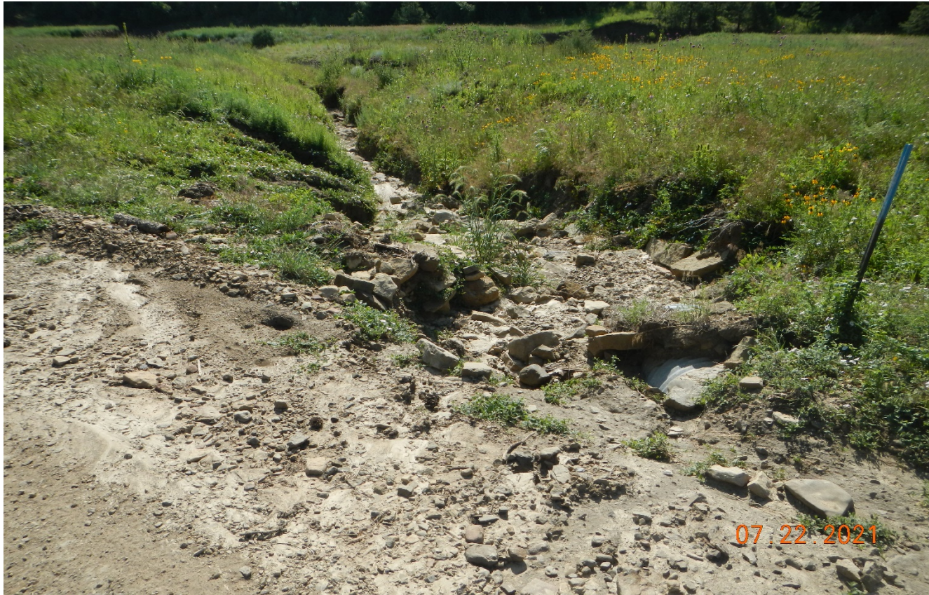
Photo 2. The culvert outlet will need to be repaired and stabilized with outlet protection.
