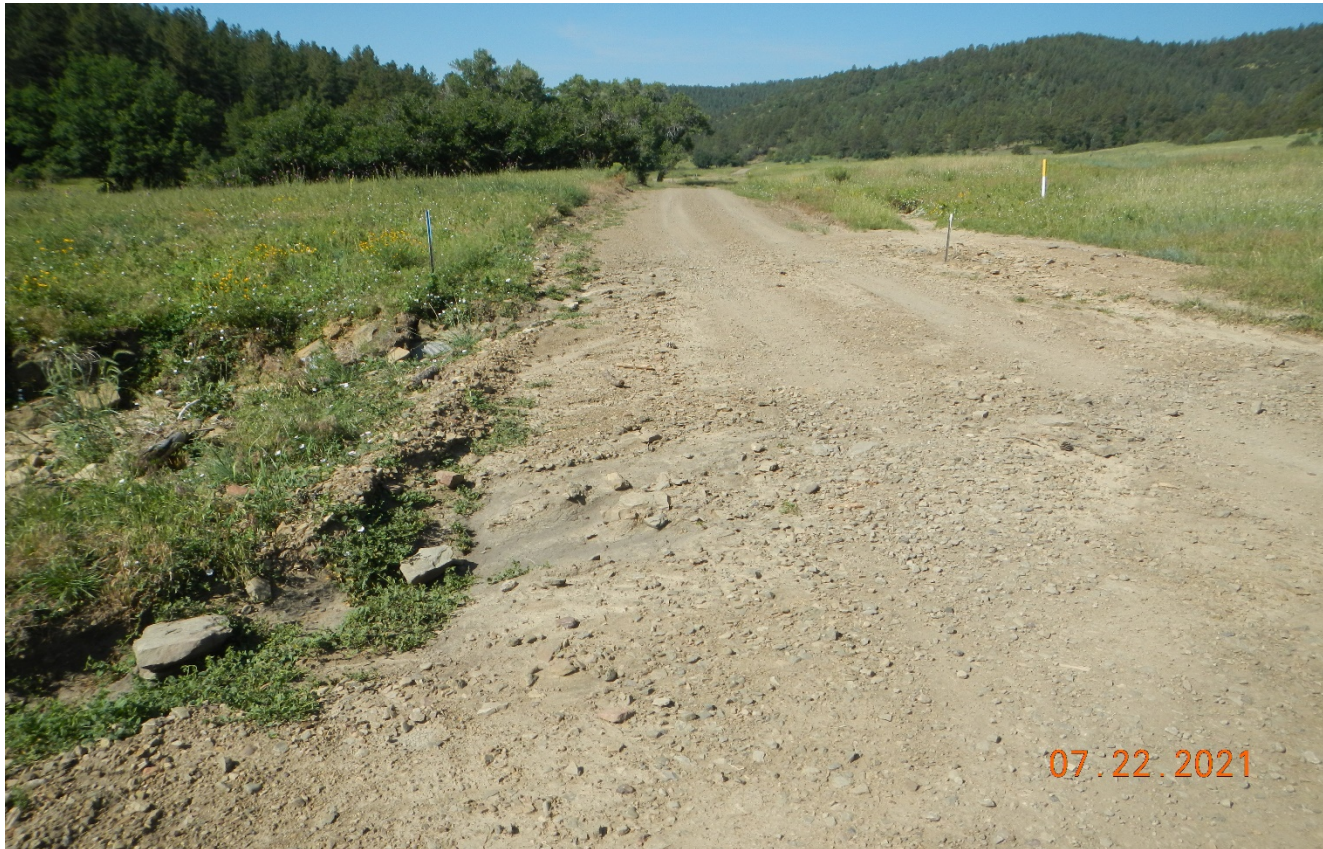
Photo 1. Facing southwest along the made road near the well site. Stormwater has washed across the road causing erosion. The culvert is filled in with sediment.
