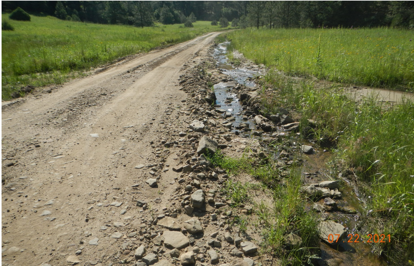
Photo 2. The culverts along the road are filled in with sediment causing stormwater to flow down the side of the road. Lat/Long:37.00499,-104.83742.
