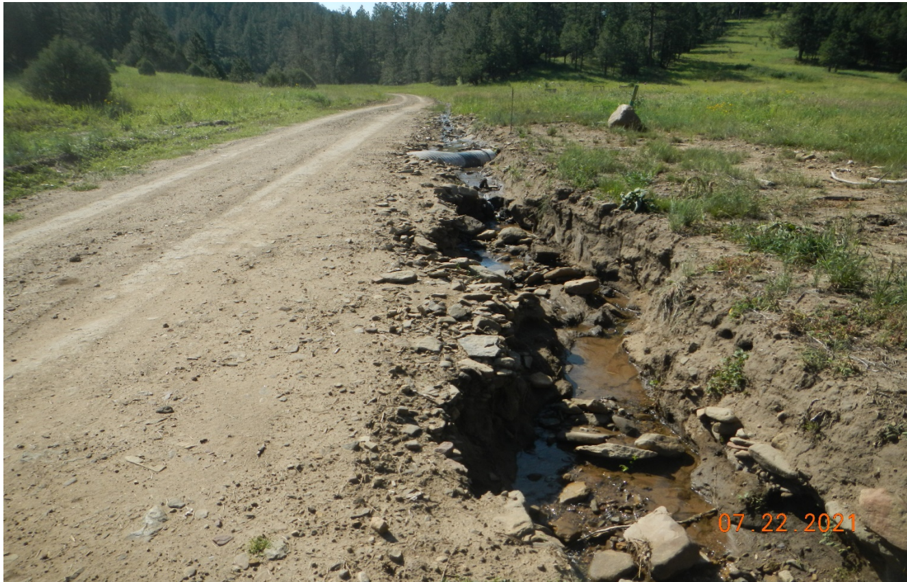
Photo 1. Facing southeast along the made road at the upper part of Lorencito Canyon. There is erosion along the road from recent storm event. Stormwater is bypassing the culvert.
