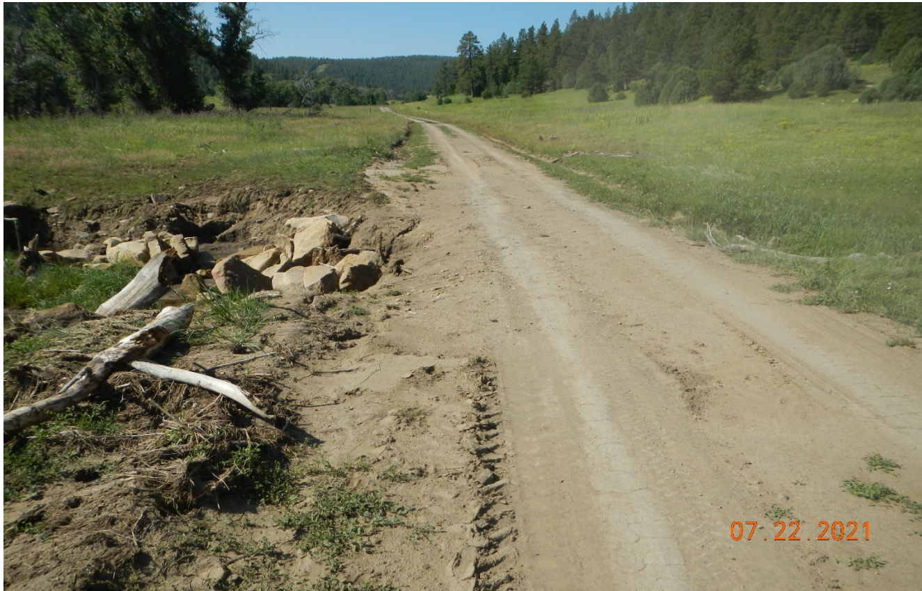
Photo 1. Facing southwest along the main road in the canyon. Stormwater has washed across the road causing erosion.
