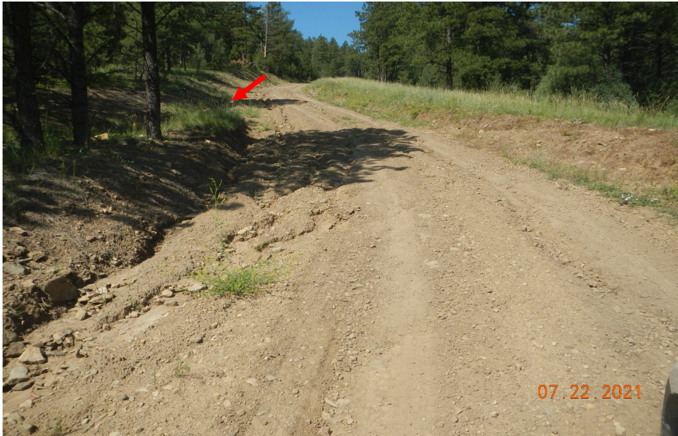
Photo 3. Facing west along the road ascending the hill toward the location. Stormwater is not properly diverted toward the ditch shown at red arrow.
