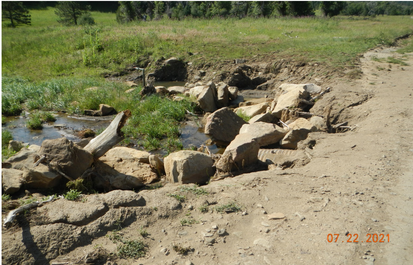
Photo 2. The culvert outlet has been eroded and will need to be repaired.
