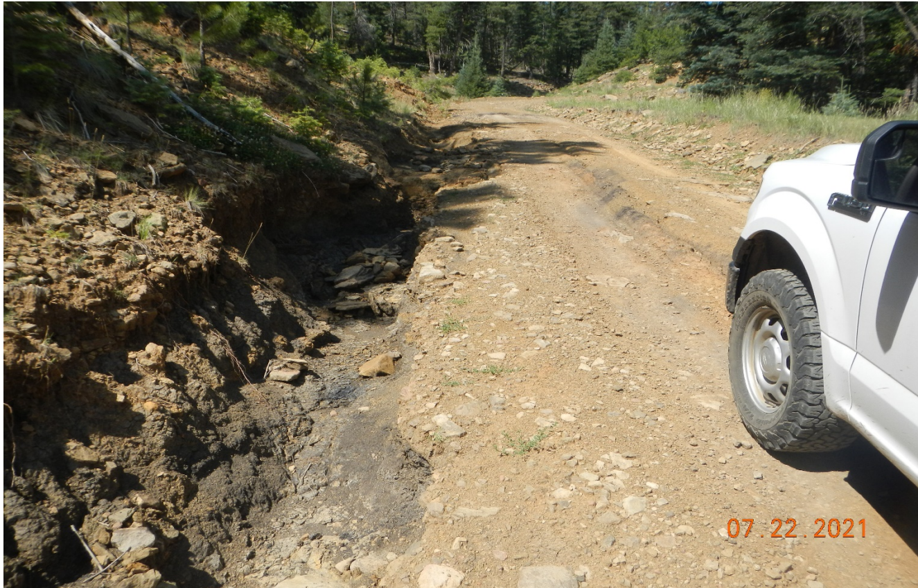
Photo 4. There is erosion along the side of the road which will need to be repaired and stabilized.
