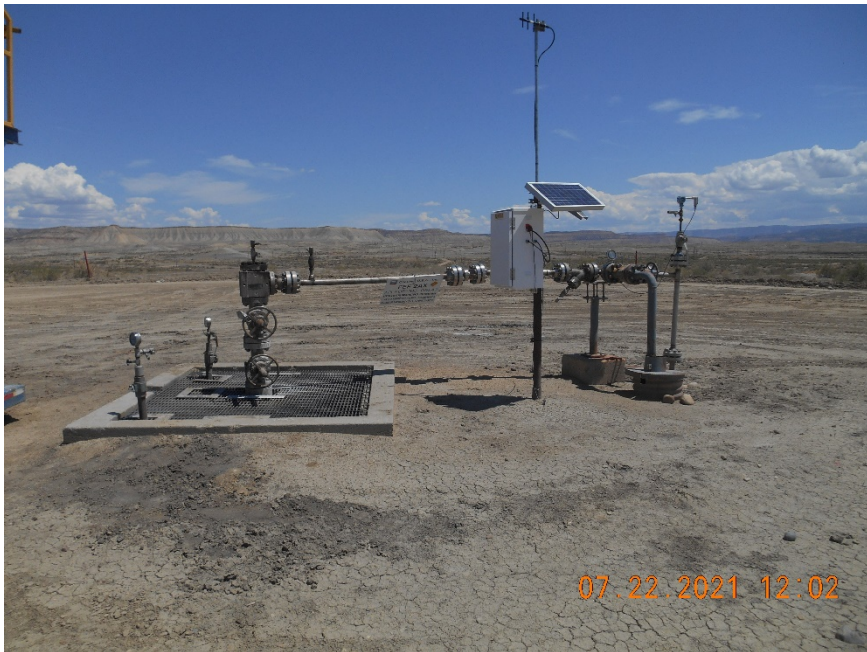
Injection wellhead
