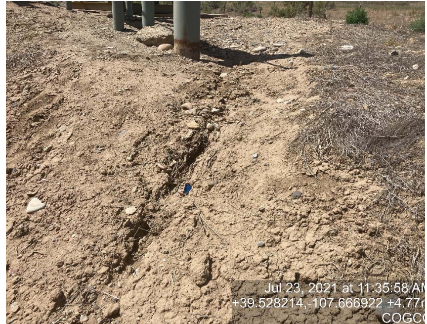
Inspection photo from most recent inspection Erosion at pig station.
