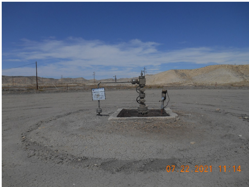
Injection wellhead.
