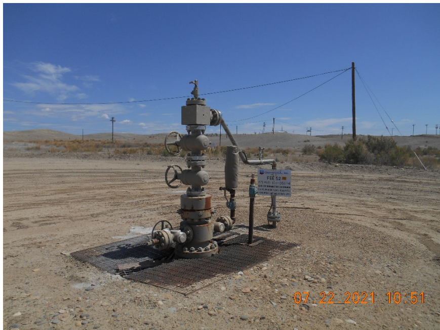
Injection wellhead.
