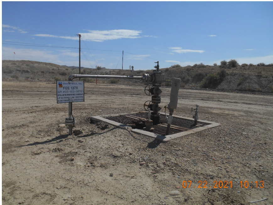
Injection wellhead
