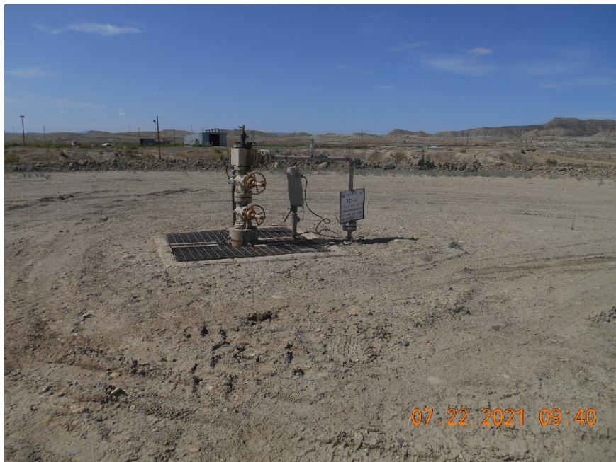
Injection wellhead.
