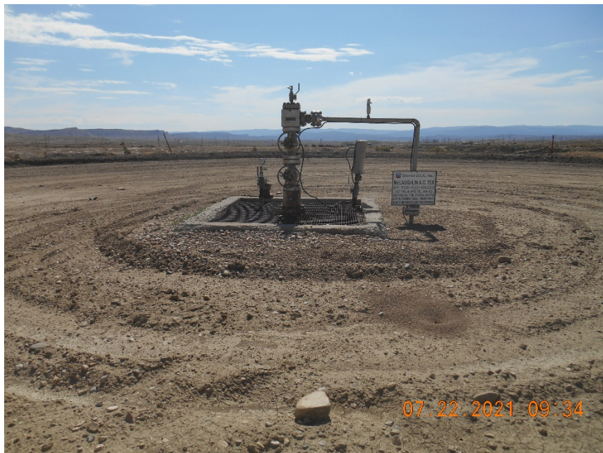
Injection wellhead.
