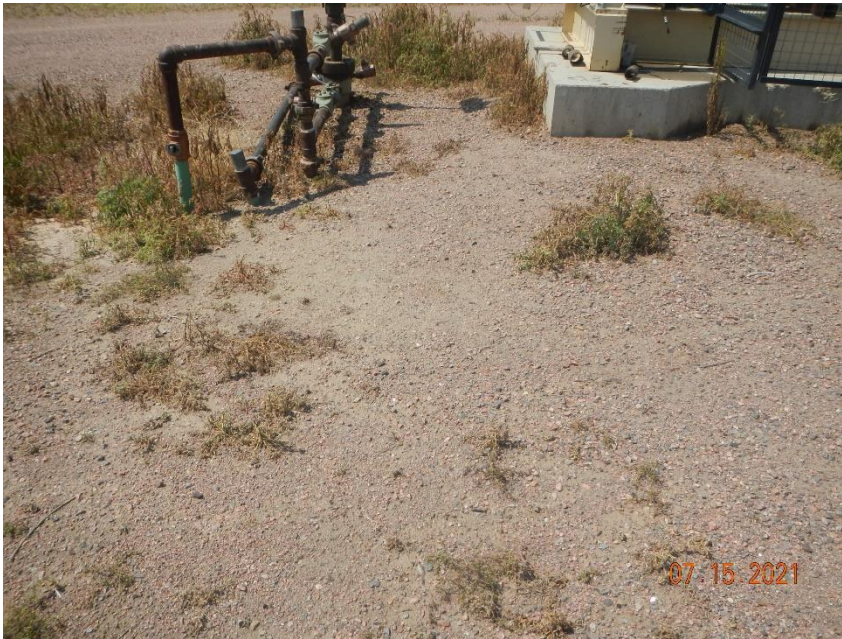
No breardenhead access, debris (dry dead weeds) around wellhead
