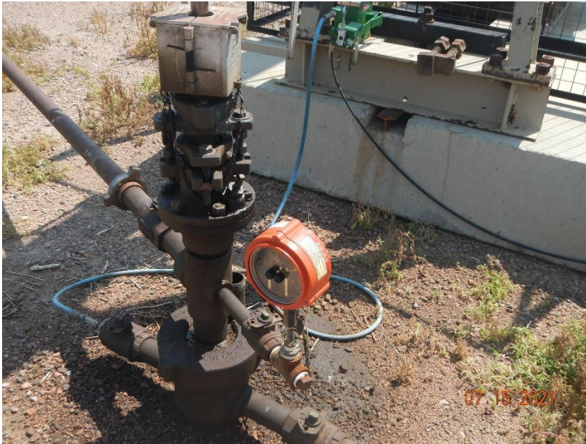
No breaddenhead access, stained soils/impacted material around wellhead
