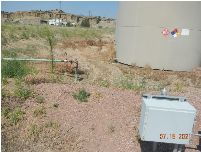
Dead vegetation debris/combustible material in containment berms, no battery sign, only DOT placard for contents labelling
