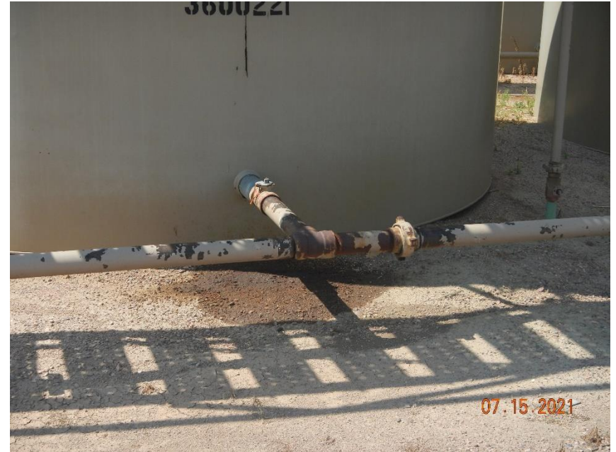
Leak/impacted material inside containment
