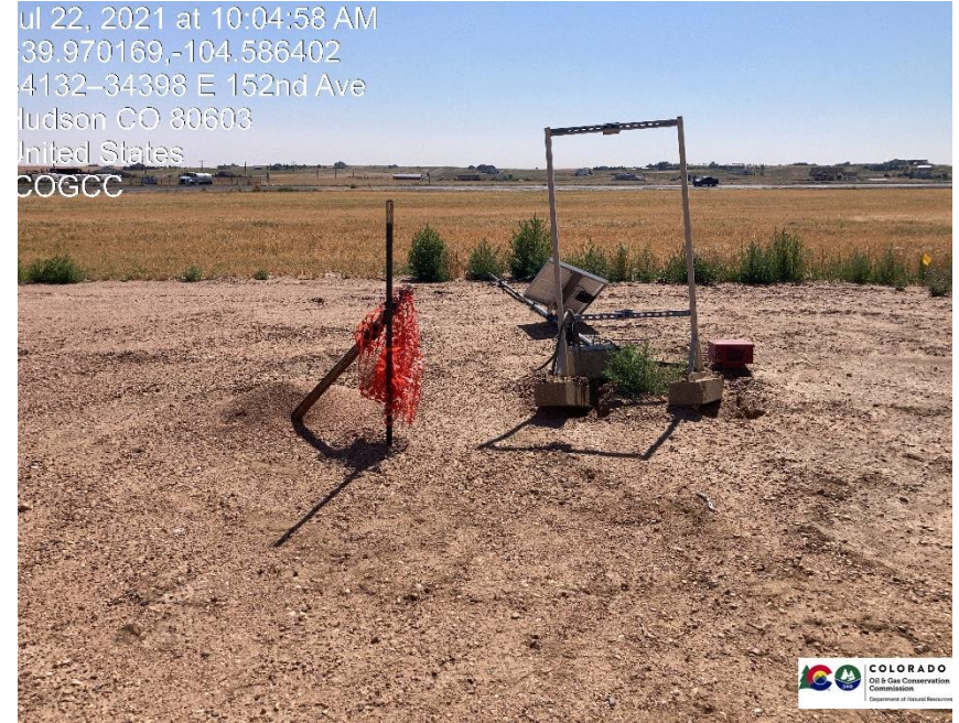
Pic 6 unused equipment
