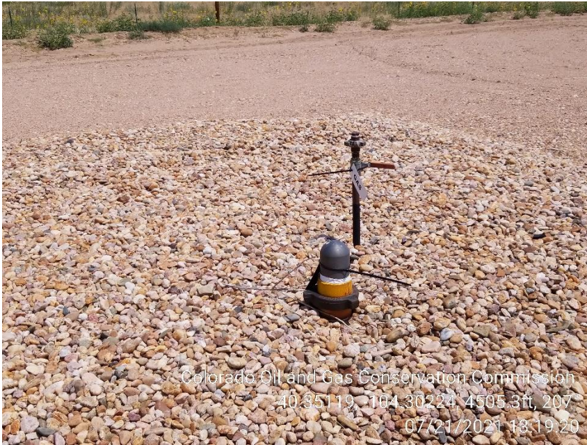
Photo 7 – Risers now marked
