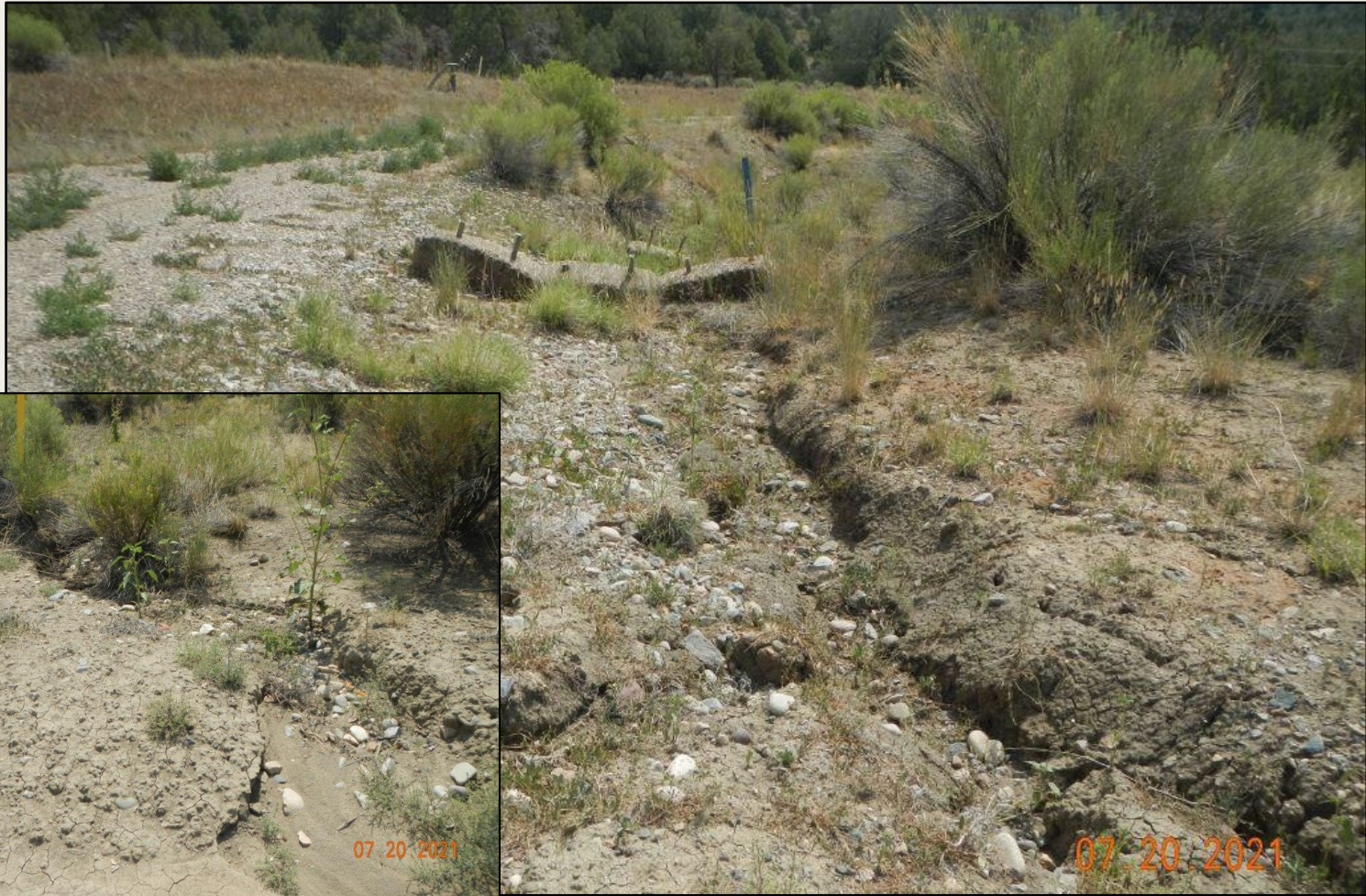
Photo 3. View of erosional rilling and channeling occurring along the access road. Straw bales are not functioning and are not an adequate BMP in this area. Inset shows erosional channeling from eroded berm on fill slope.
